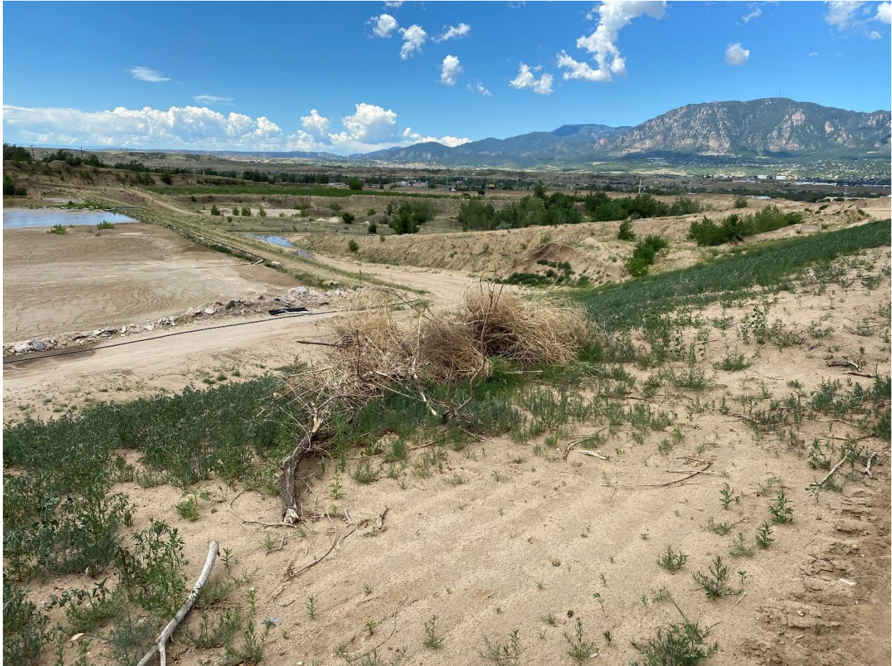
Photo 5. Buttress slope with branches
