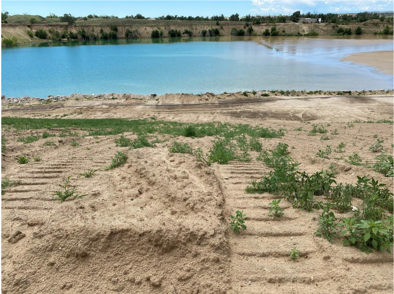
Photo 9. Buttress slope looking south, area needs regrading
