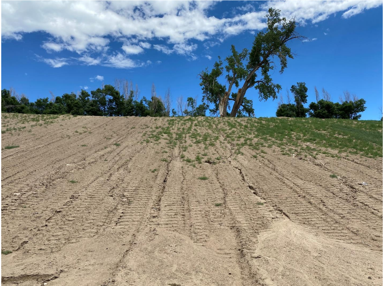
Photo 8. Buttress slope looking north, evidence of surface water drainage
