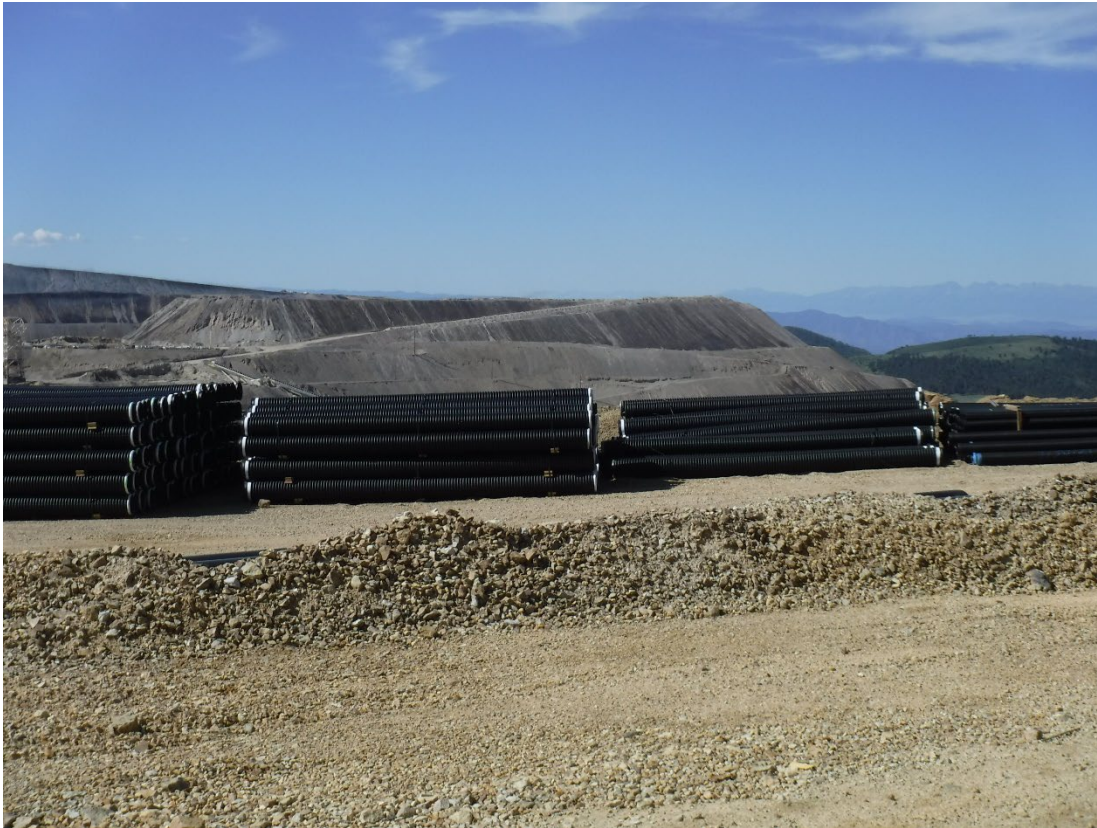
Photo 5: Staged under-drain materials near the warehouse area in preparation for deployment
