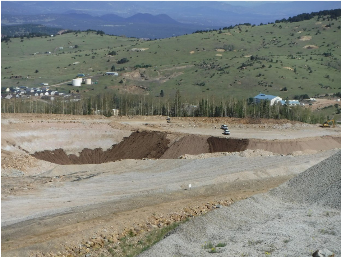
Photo 3: Placement of the clay base layer in preparation for liner material
