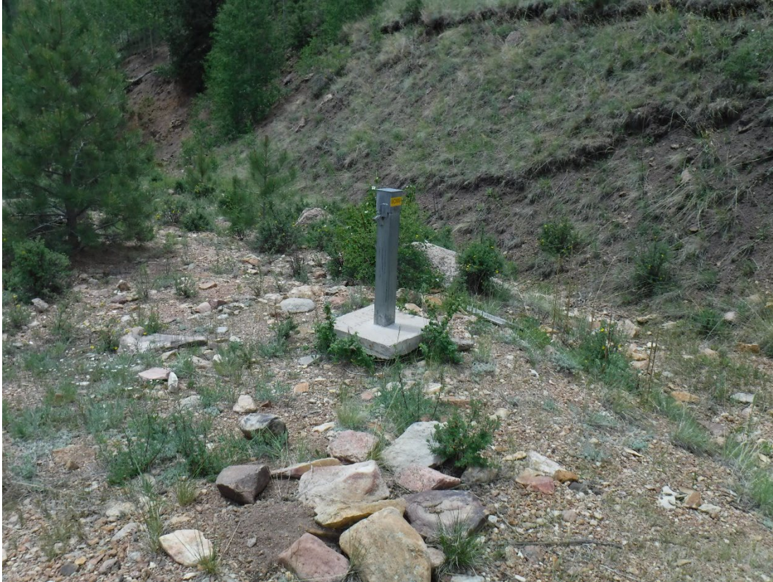
Photo 9: WCMW-6, note vegetation growing up from underneath the concrete pad
