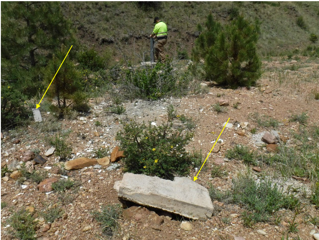
Photo 10: WCMW-6 in the background, arrows point to broken concrete pad and 1 of 3 discarded protective casings
