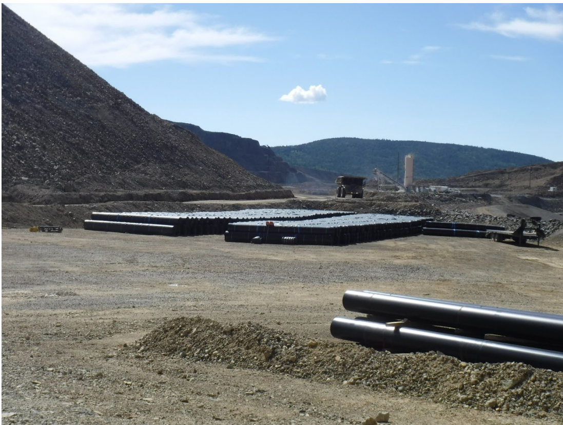
Photo 4: Staged liner material near the warehouse area in preparation for deployment
