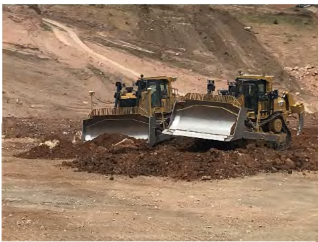
5. Dozers spreading material placed in the pit area.
