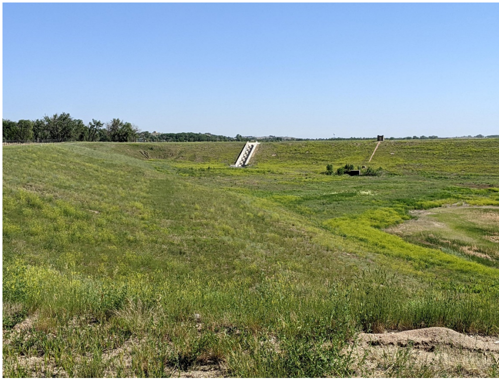
Looking north at overflow drain between Reservoir A & B. Flood repair occurred on western slopes.
