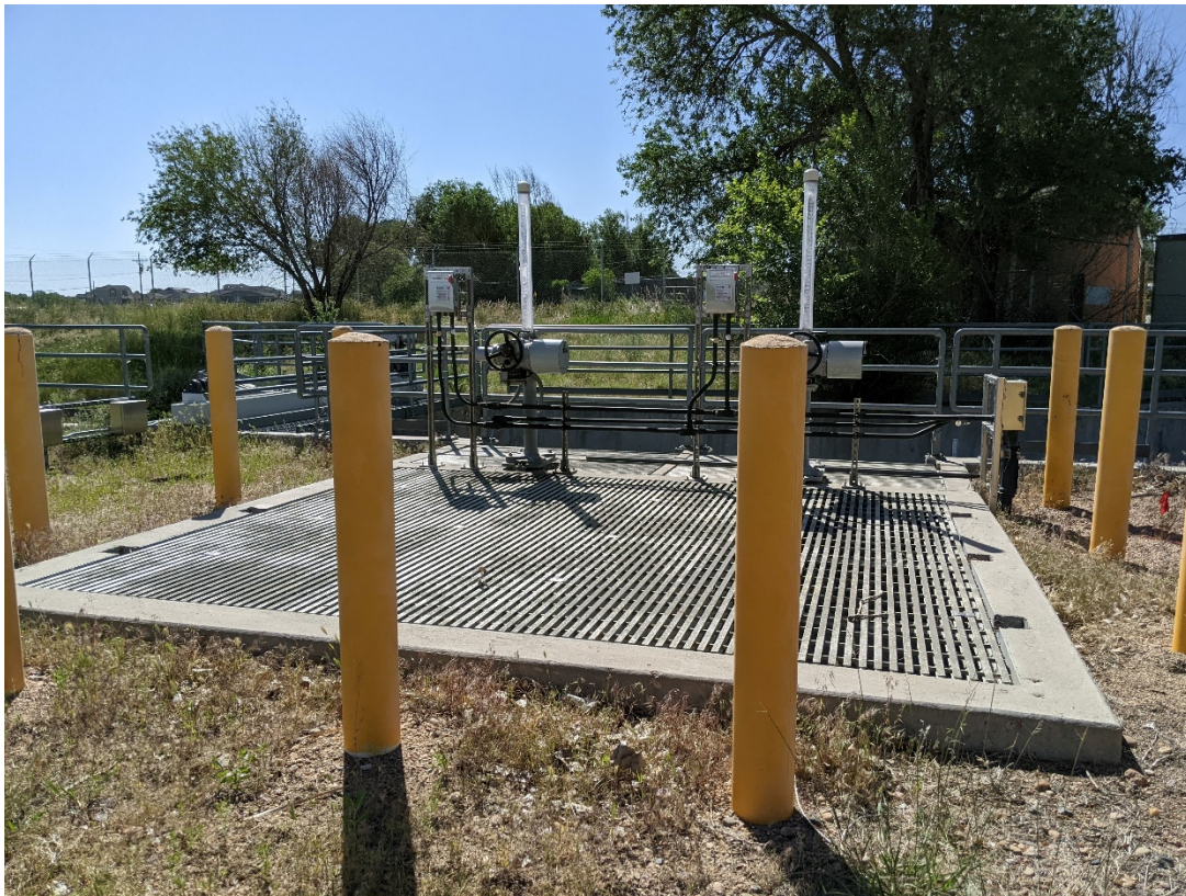
Headgate and monitoring station on irrigation canal east of Reservoir A.
