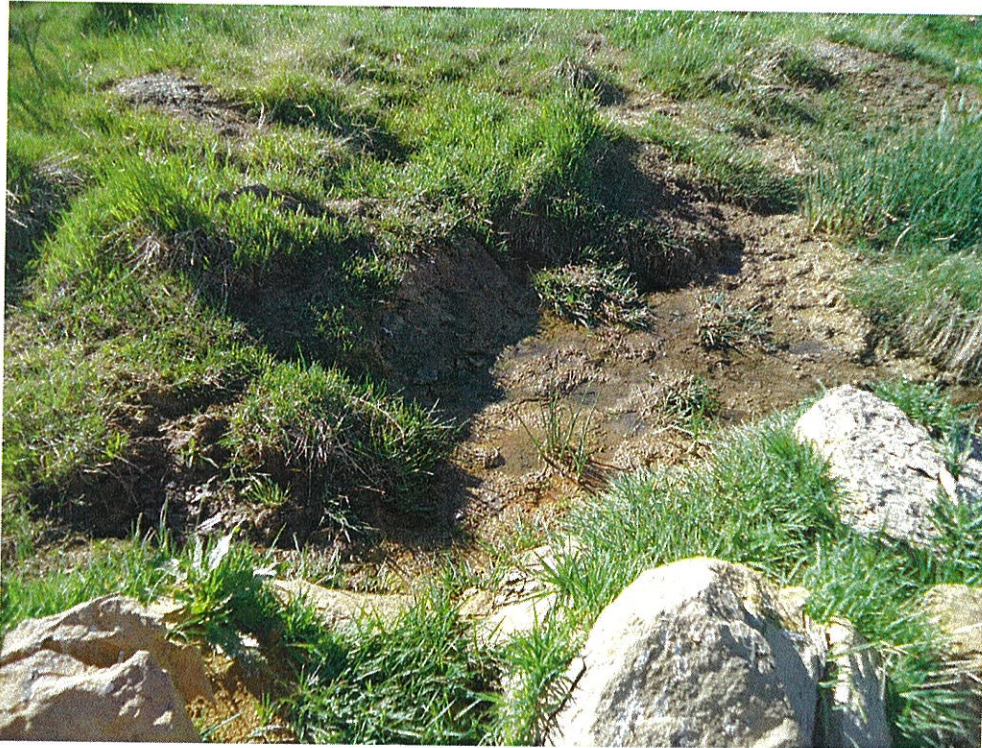
Photograph 5: Water from the Underdrainage System (6/15/2022)
