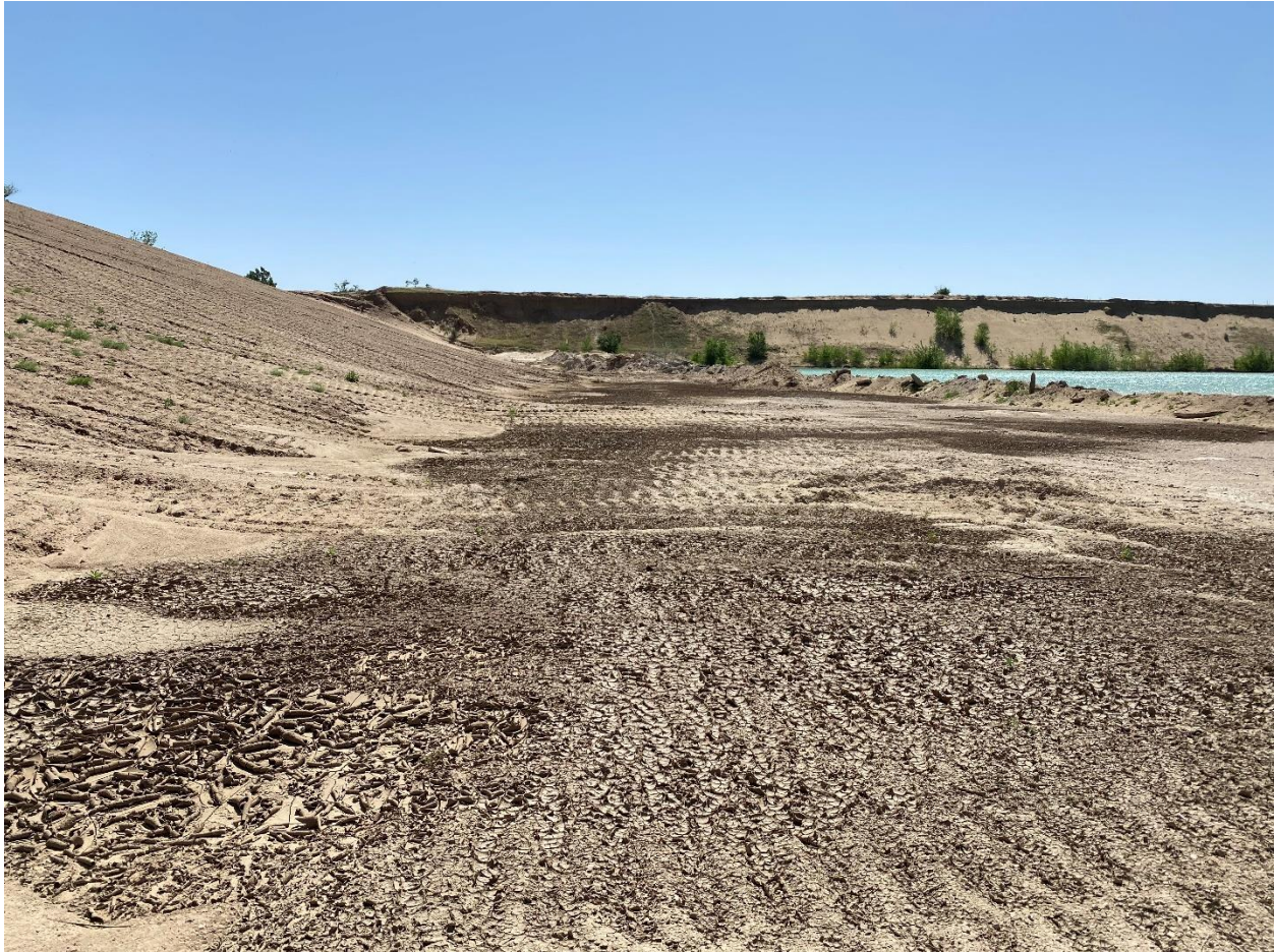
Photo 11. Evidence of previous ponding water near toe of buttress
