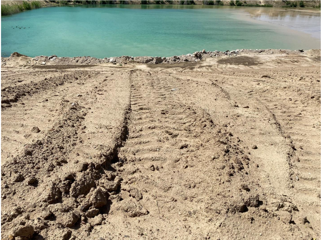
Photo 9. Butress slope looking south, area needs regrading
