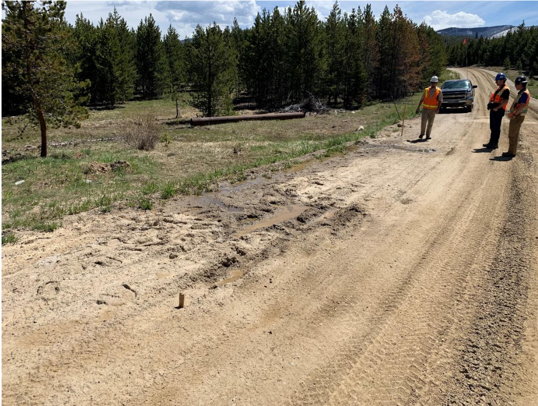
Photo 9 – Water expression along west access road, facing southeast, the leaky valve is just beyond the trees above the truck
