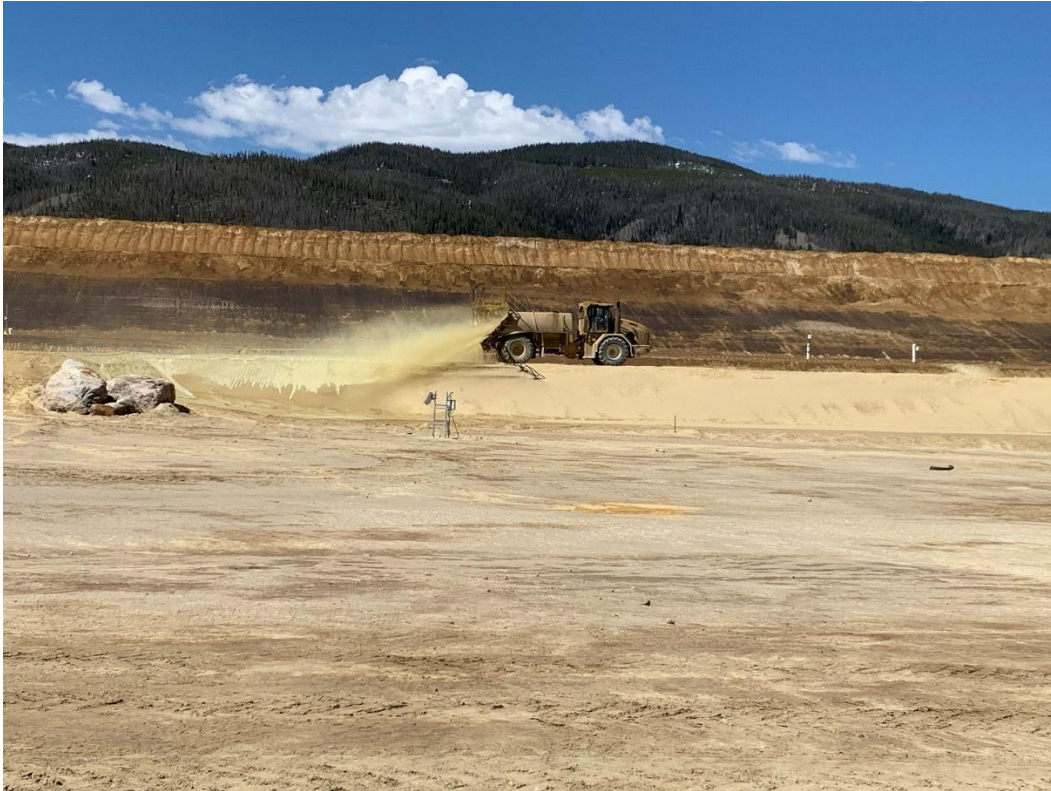
Photo 3 – Coherex application on 3-Dam
