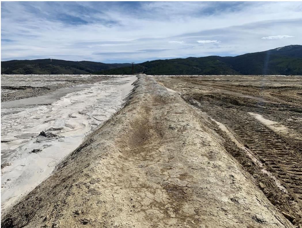
Photo 1 – Top of TSF, tailing are sandy and whitish/grey, no Coherex applied
