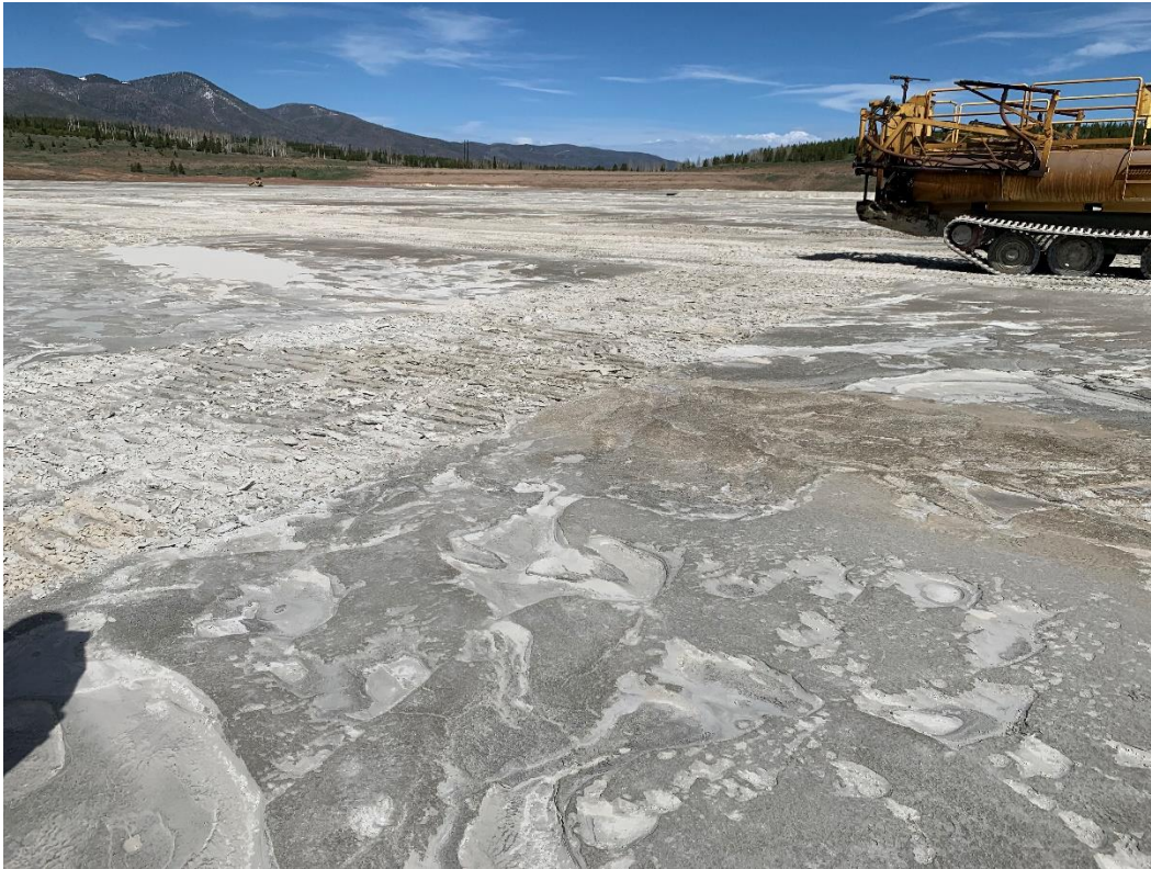
Photo 1 – Top of TSF, tailing are sandy and whitish/grey, no Coherex applied
