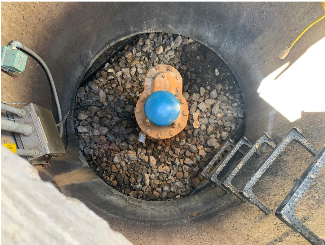
Photo 8 – Leaky vent valve on the Mill Water Return Line
