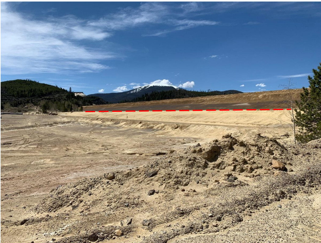
Photo 4 – Coherex applied above dashed line
