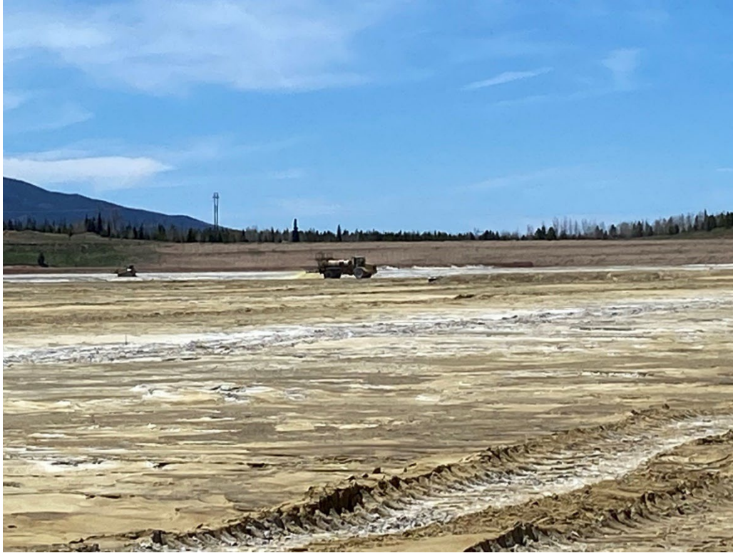
Figure 4. Coherex spray truck on the tailings beach applying Coherex on May 16 th (a) and 27 th (b).
