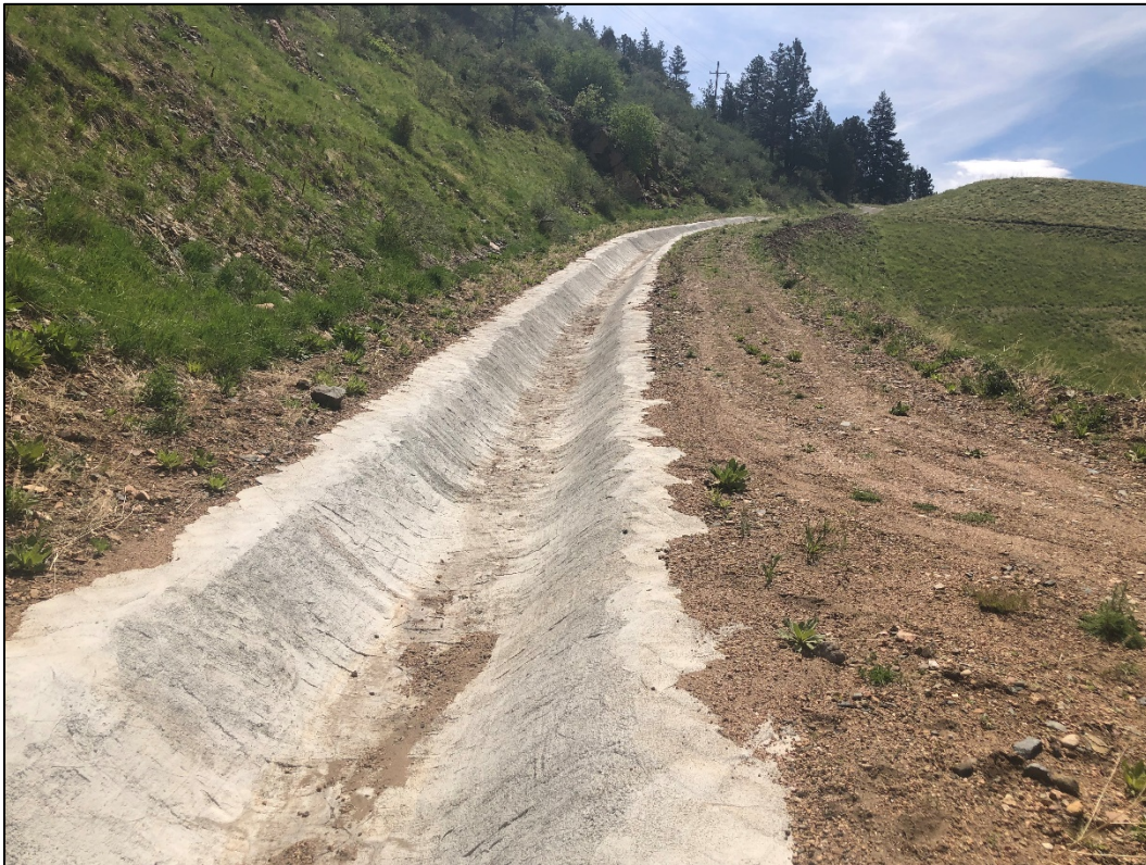
Photo 10. View looking upgradient at diversion channel installed along northern edge of NWRP in 2020.
