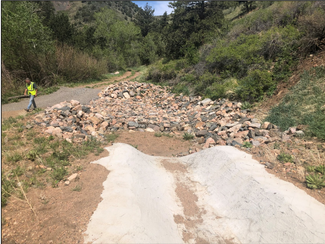
Photo 11. View looking west at riprap-lined energy dissipation basin constructed at downgradient end of NWRP diversion channel. This basin should be kept free of sediment and vegetation.
