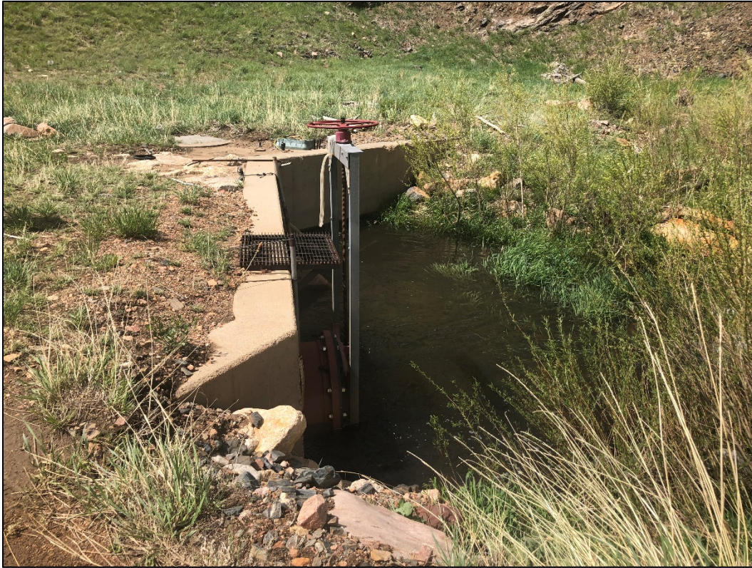
Photo 9. View of upgradient cutoff wall/headgate in Ralston Creek, showing creek flowing upstream of cutoff wall. Upgradient flows were being routed around the mine site via the bypass pipeline.
