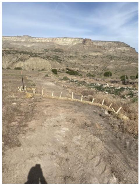
The straw waddle in the photo above was replaced during the inspection. The straw waddle in this location was damaged when the landowner scraped the surface through the TR-69 repair area. The scrapped path was similar to the inspections conducted earlier in the week.
