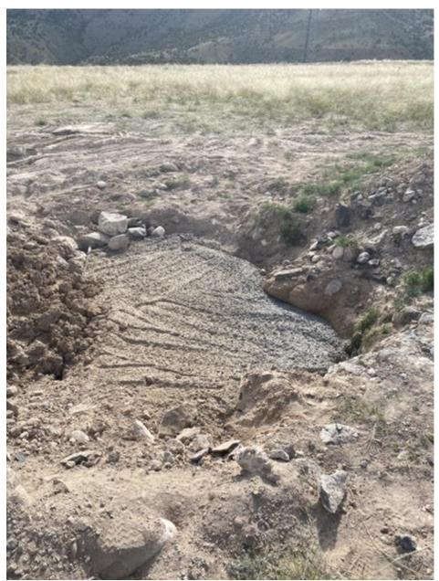
The photo above was taken of the cement cap located on top of the Tract 70 Mesa. The hole with the cement in it was approximately 3 feet by 4 feet.
