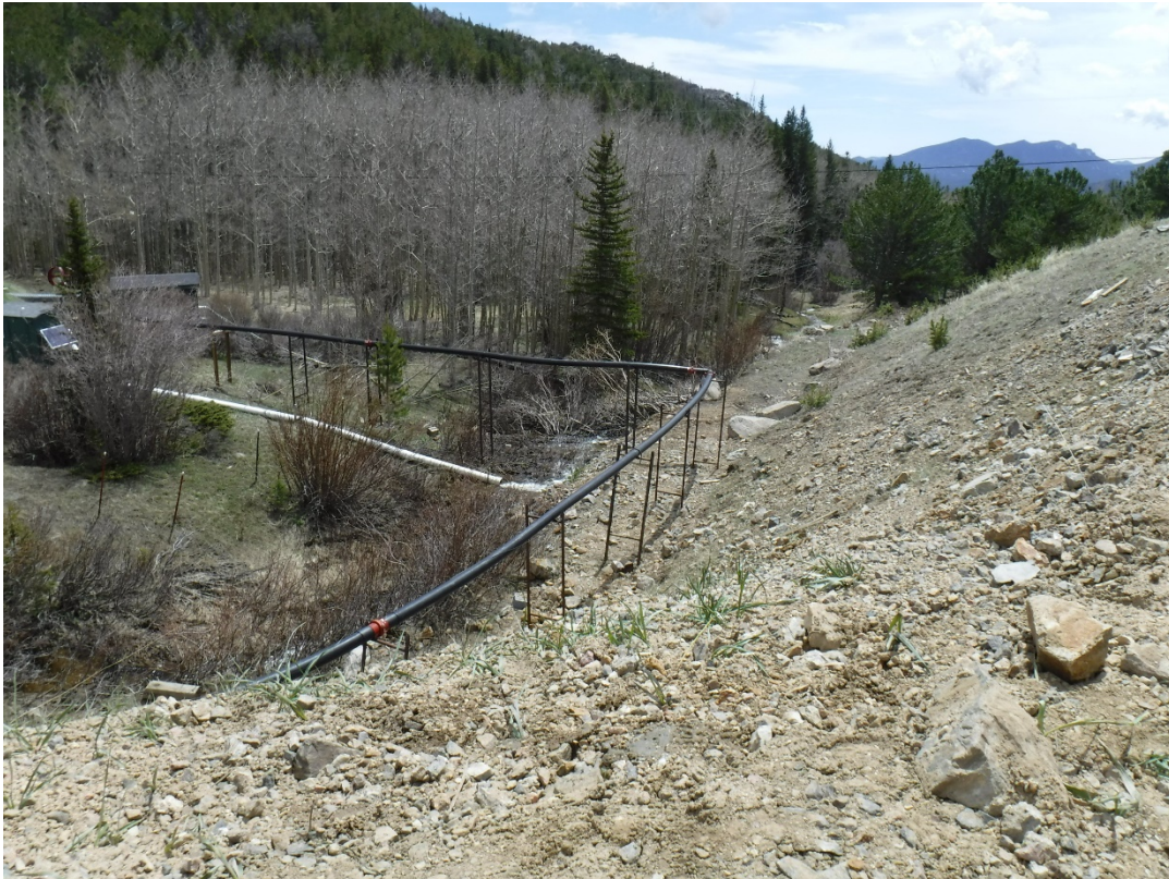
Photo 6: Elevated pipeline that goes from the water treatment to the discharge shed then to the WQCD discharge point to Coon Track Creek
