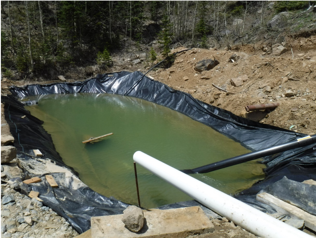
Photo 16: Pond 3a, first settling pond receiving effluent from the Caribou Mine
