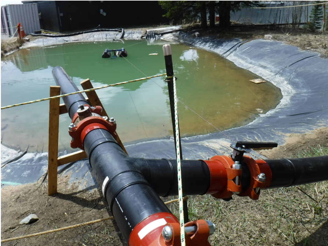
Photo 10: Pond 1 showing the outfall from Pond 3c, the T-fitting directs flow to Juliet Raise during high runoff
