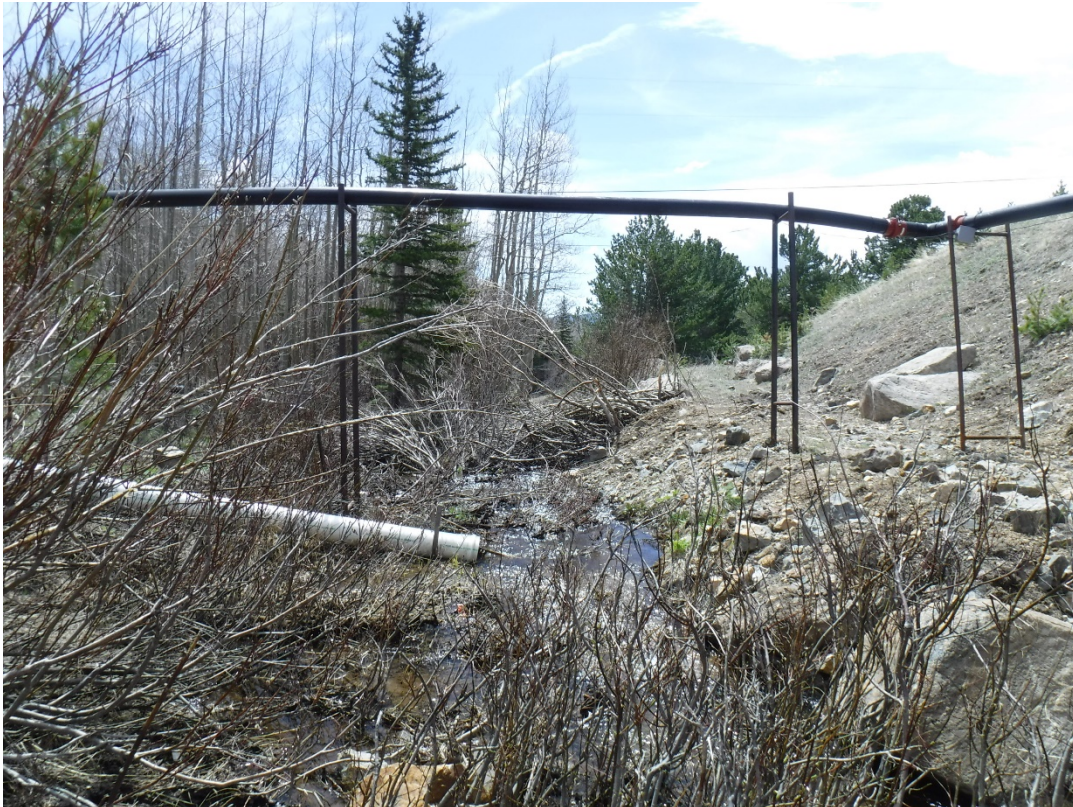
Photo 8: Permitted discharge point to Coon Track is at the outfall from the white PVC pipe
