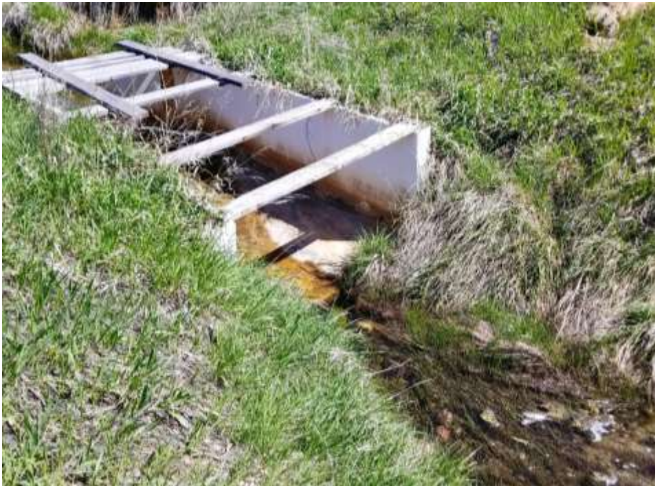
Below: Flume being undercut
