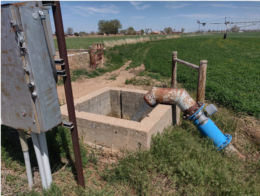
View of the inlet vault from the well to the irrigation system
