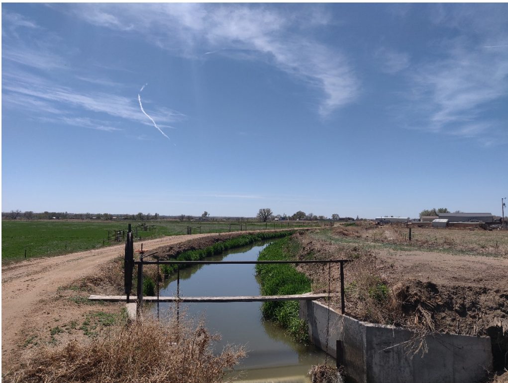
View of the Lupton Meadows Bottom Ditch located west of the well
