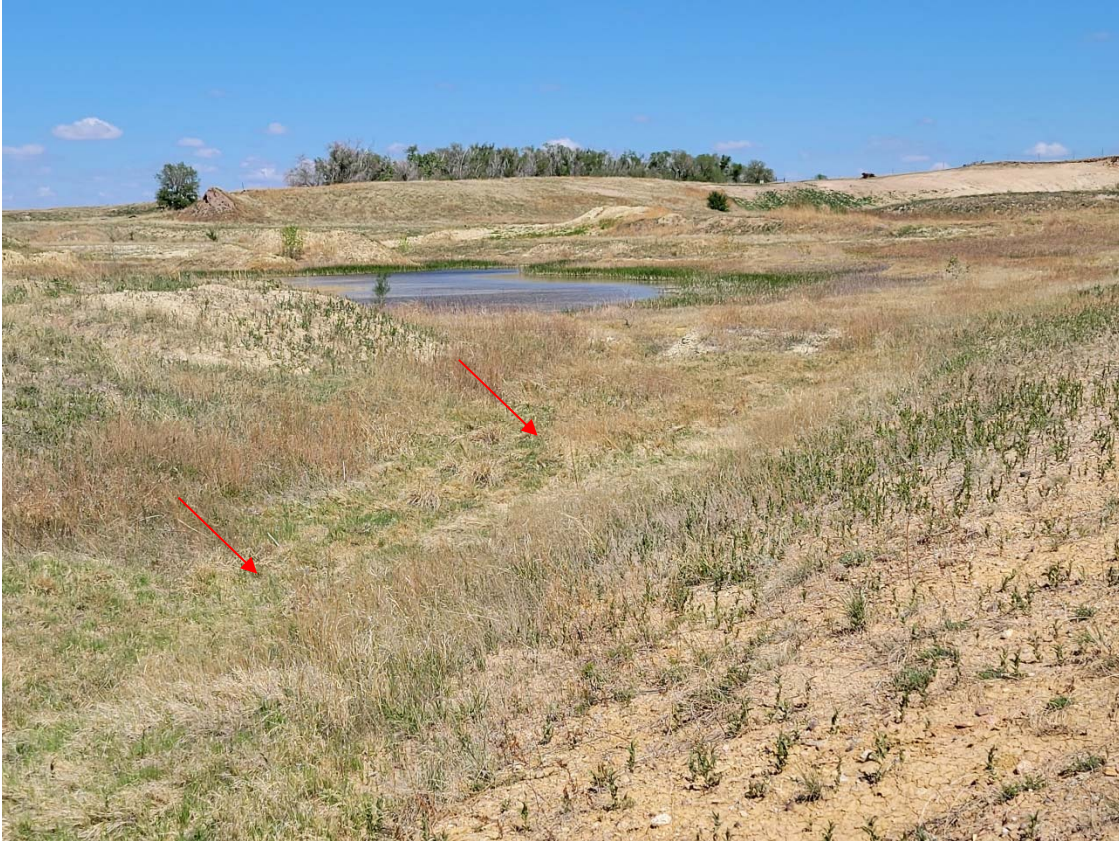
Looking northwest. Drainage ditch excavated to drain pond.
