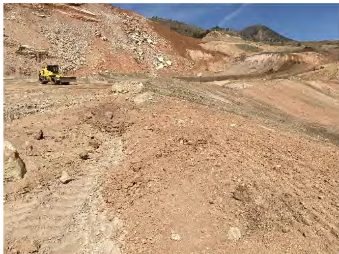
7. Compactor in the pit area.
