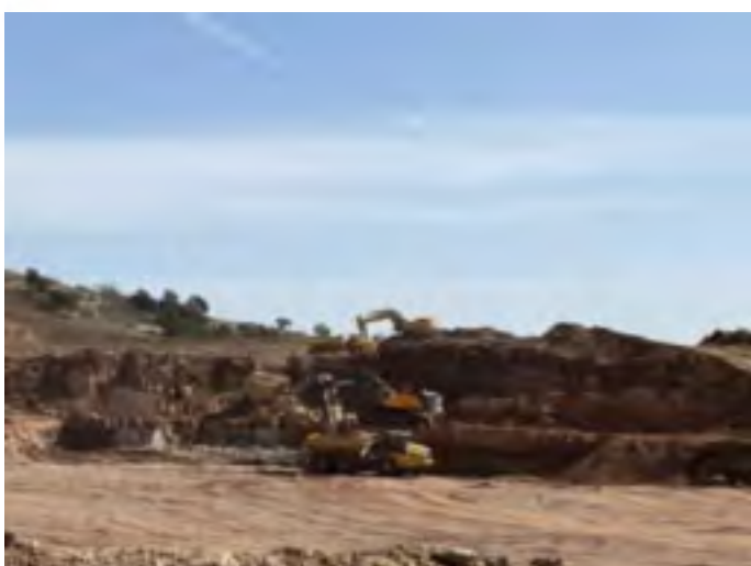
1. Excavators cutting a bench in the North Borrow area.
