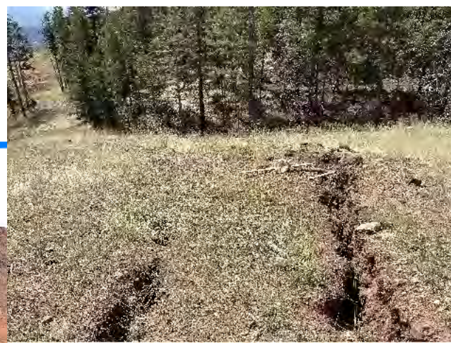
4. Old cracks being monitored on the south end.
