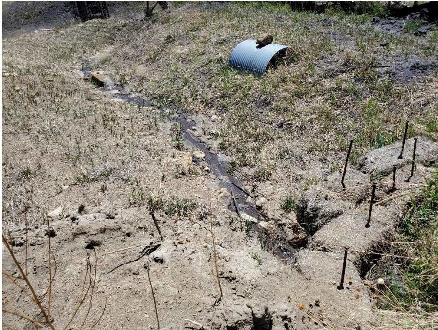
Figure 11. Drainage ditch section that connects to Containment Area 5 immediately east of the conveyor that needs to be enhanced.
