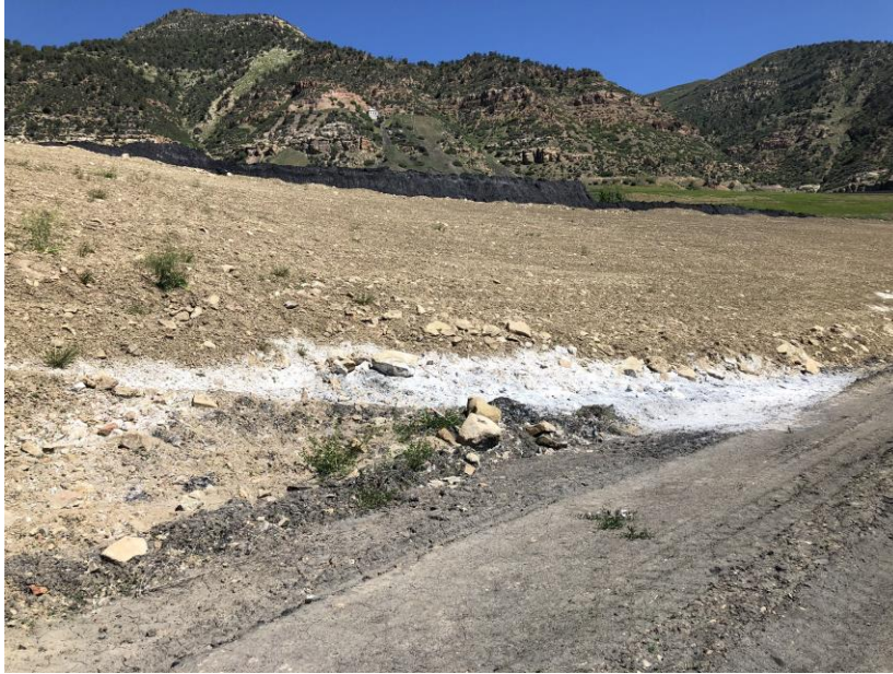
Evidence of leachate through Gob Pile #3
