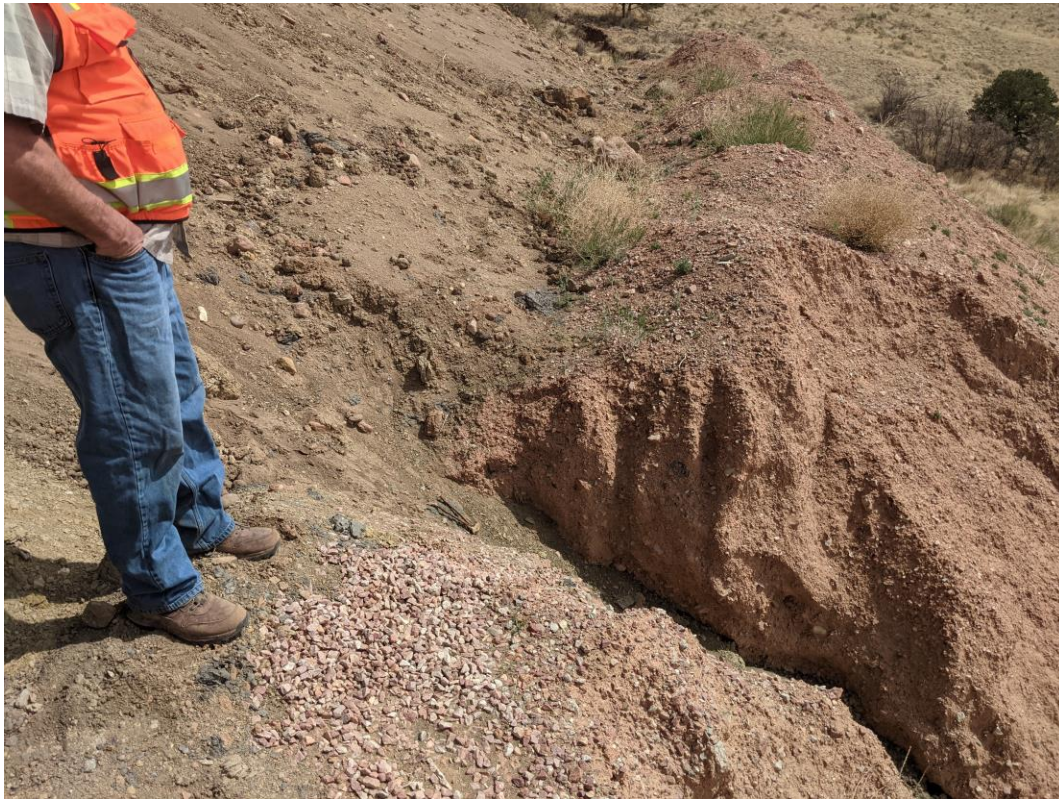
Photo 1. Erosion along topsoil pile berm.
