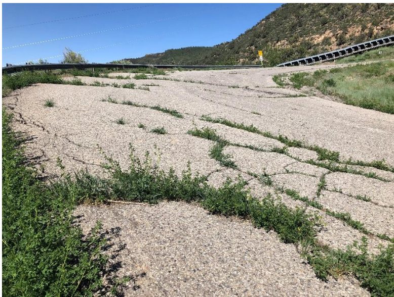
Cracks on road to portals (Curve 5)
