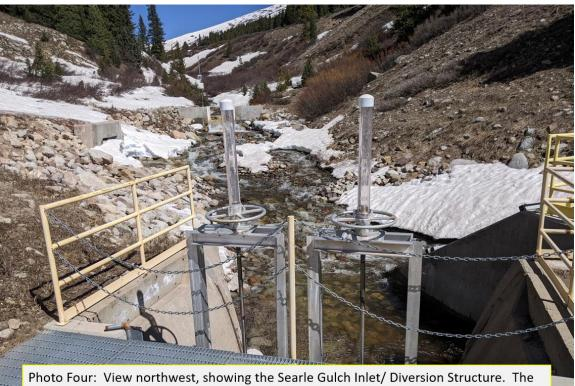
Photo Four: View northwest, showing the Searle Gulch Inlet/ Diversion Structure. The structure is in excellent condition and functioning as designed. At the time of Inspection, all flow was being directed into the West Interceptor.
