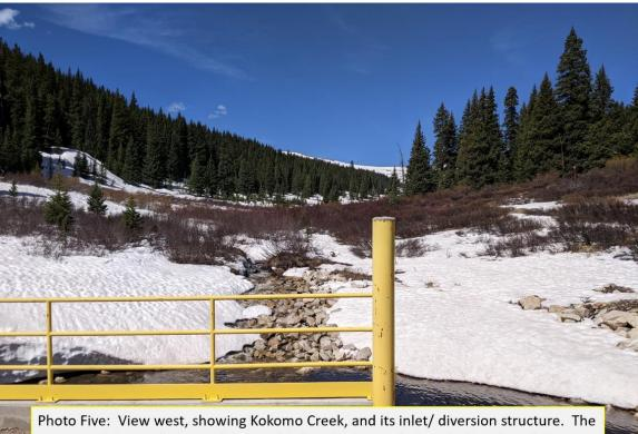
Photo Five: View west, showing Kokomo Creek, and its inlet/ diversion structure. The structure is in excellent condition and is functioning as designed, diverting all flow from Kokomo Creek into the West Interceptor.
