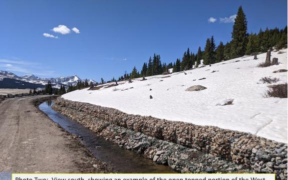
Photo Two: View south, showing an example of the open topped portion of the West Interceptor Ditch. This section has had the upgradient side reinforced with Gabion Baskets that are in good condition. The entire length of the observed open topped portion of the West Interceptor is free from obstruction and flowing unimpeded.
