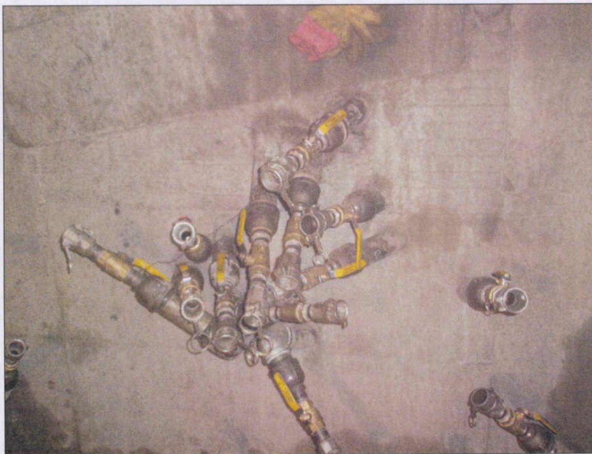
Figure 8: Typical array of contact grouting pipes
