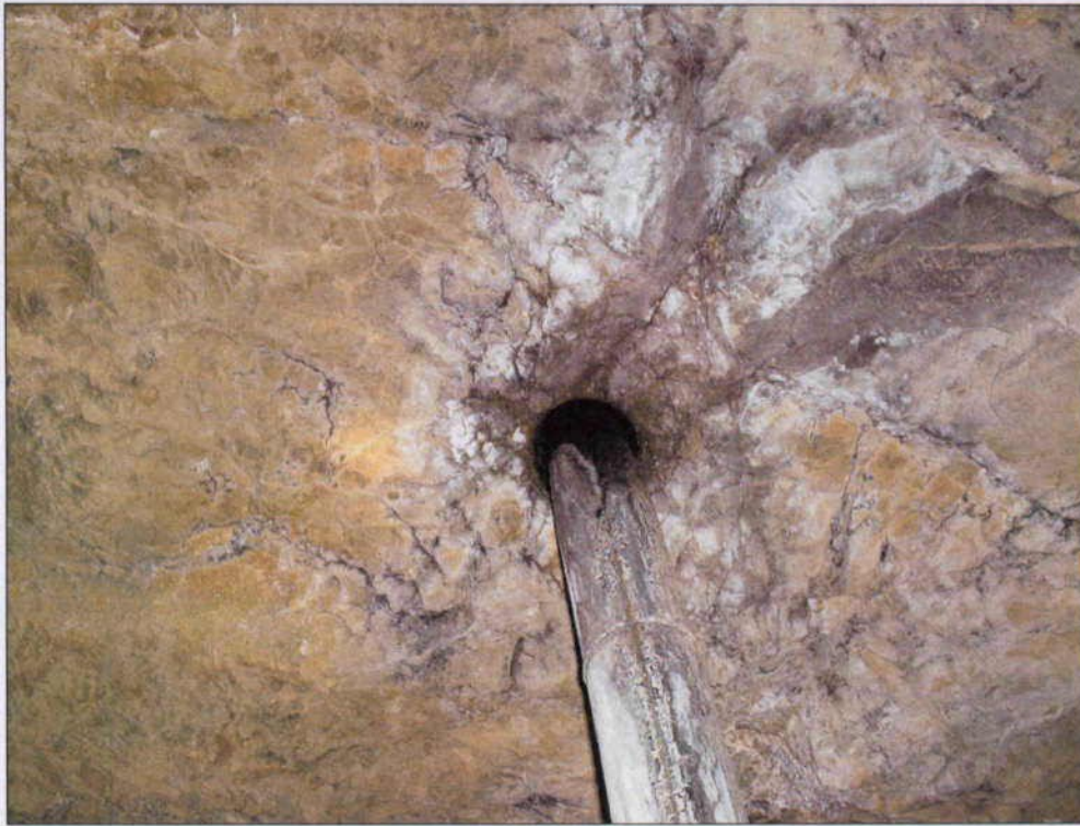
Figure 4: Borehole in Pierce adit roof
