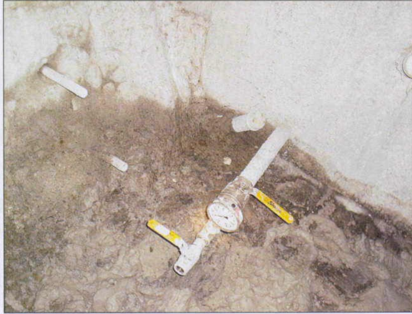
Figure 11: Typical drain valve assembly
