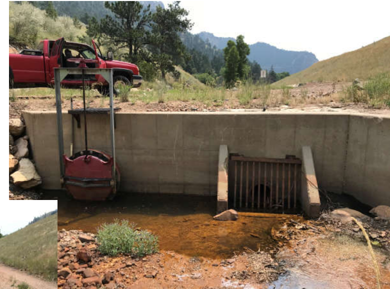
Spring 2018: Intake for Ralston Creek diversion across CLL property. Bypass pipeline and cutoff wall
