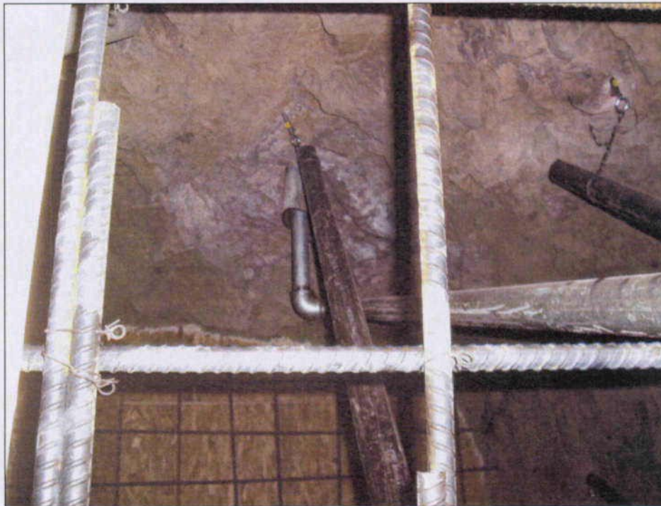
Figure 10: Placement of grout pipes for borehole abandonment
