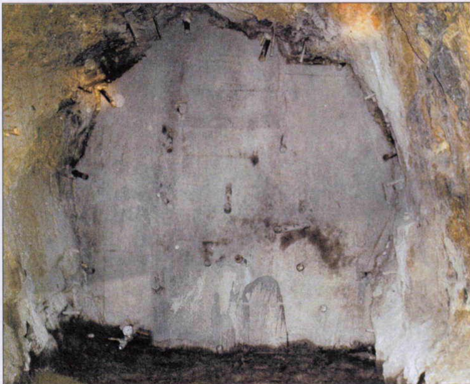
Figure 14: Completed bulkhead – Pierce adit
