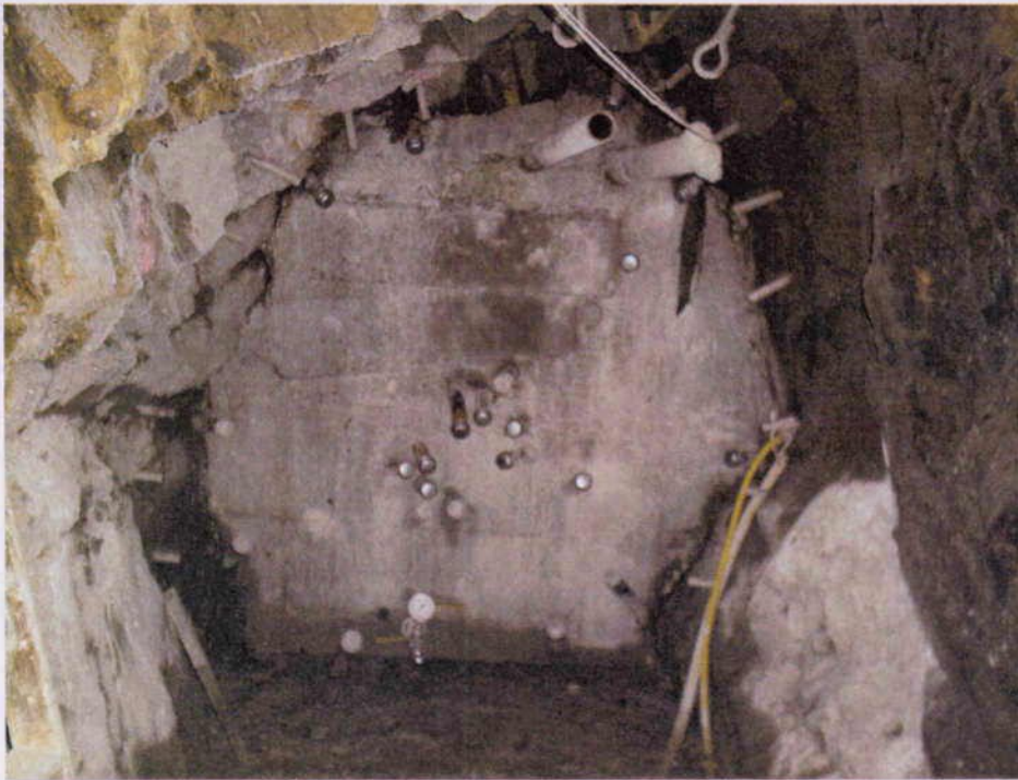
Figure 13: Completed bulkhead – Steve adit
