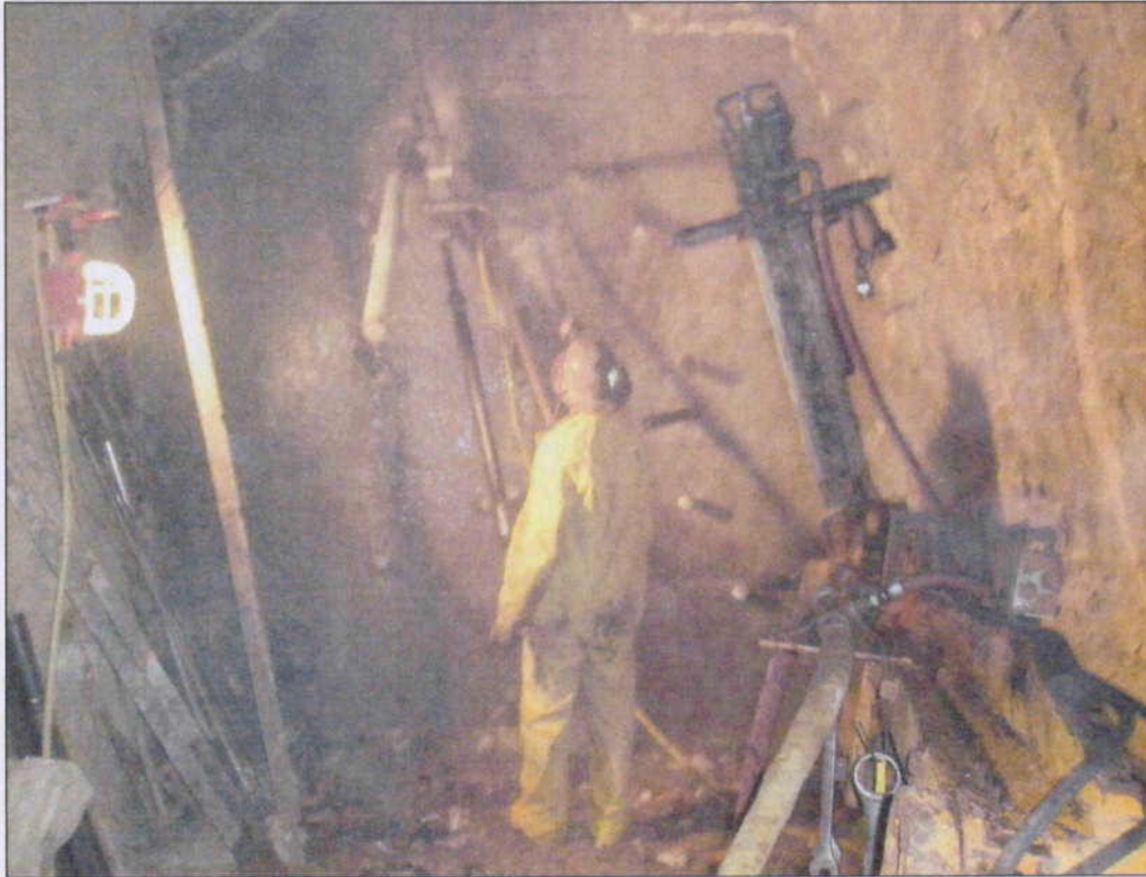
Figure 9: Grout hole drilling
