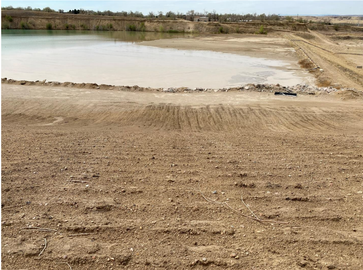
Photo 8. Buttress slope looking south
