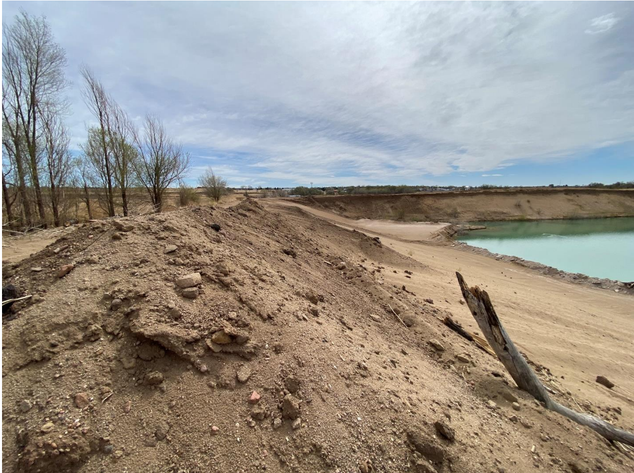
Photo 10. Buttress slope looking east, branches near stockpiled material and buttress slope
