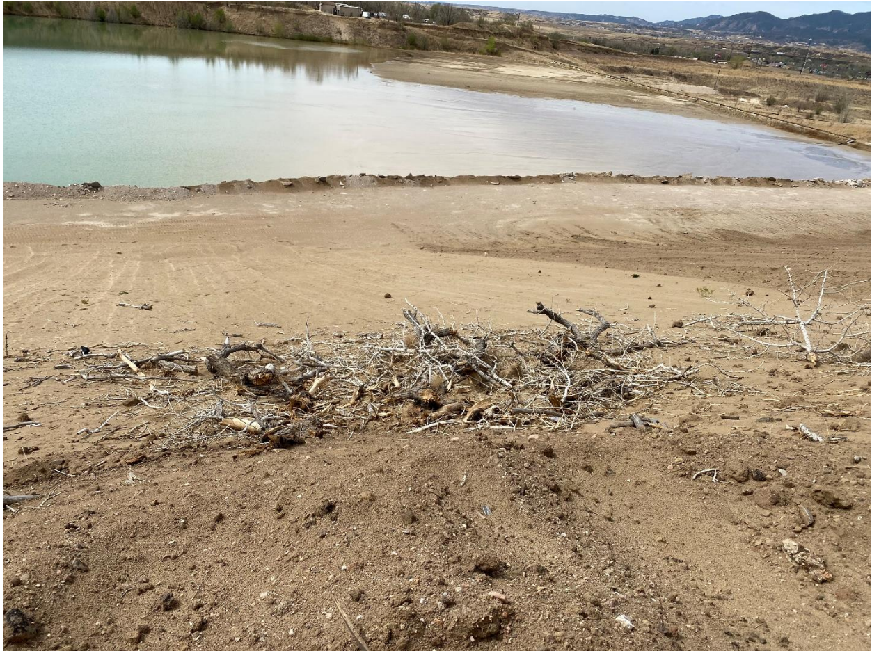
Photo 7. Butress slope looking south (note branches)
