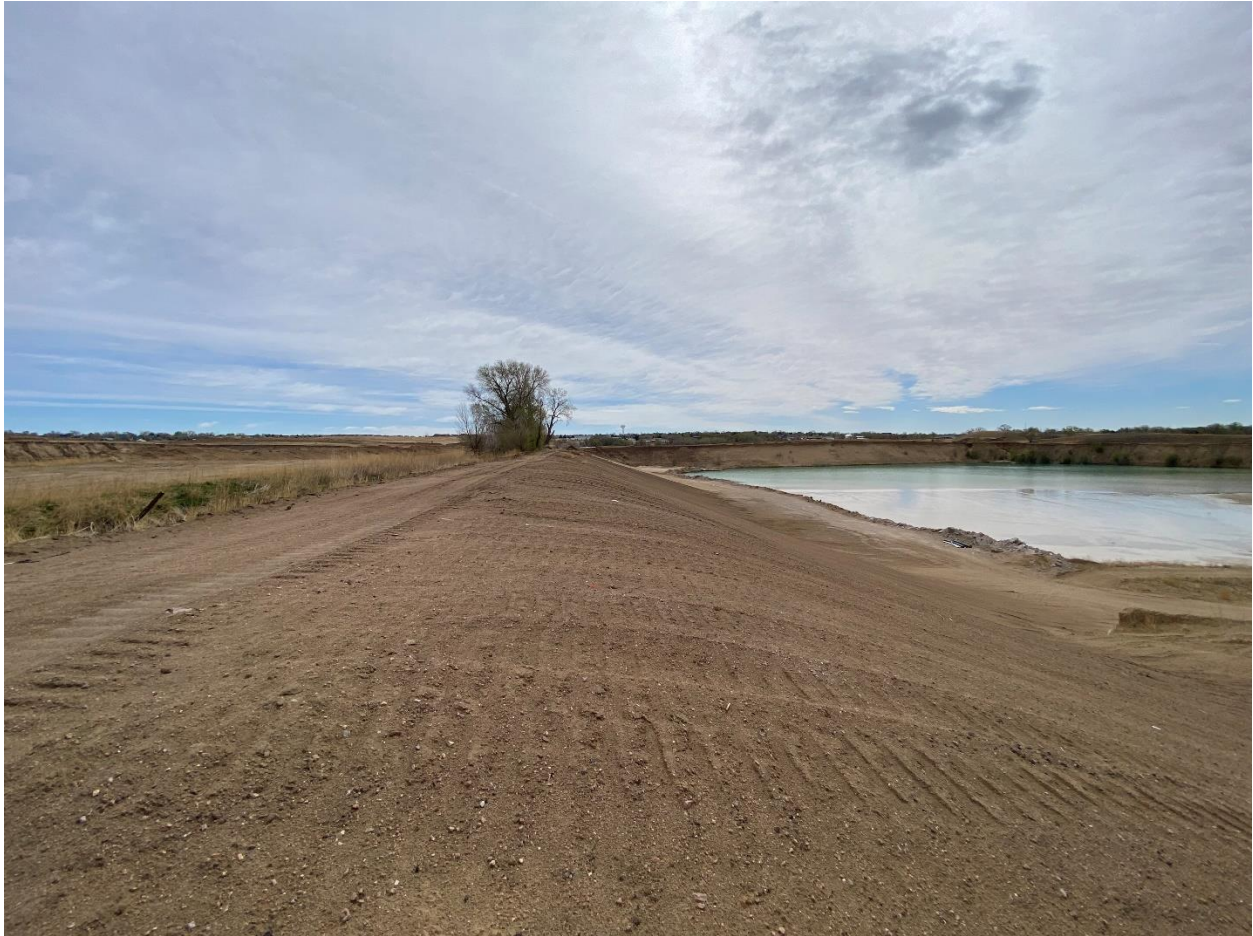
Photo 6. Buttress slope looking east from crest
