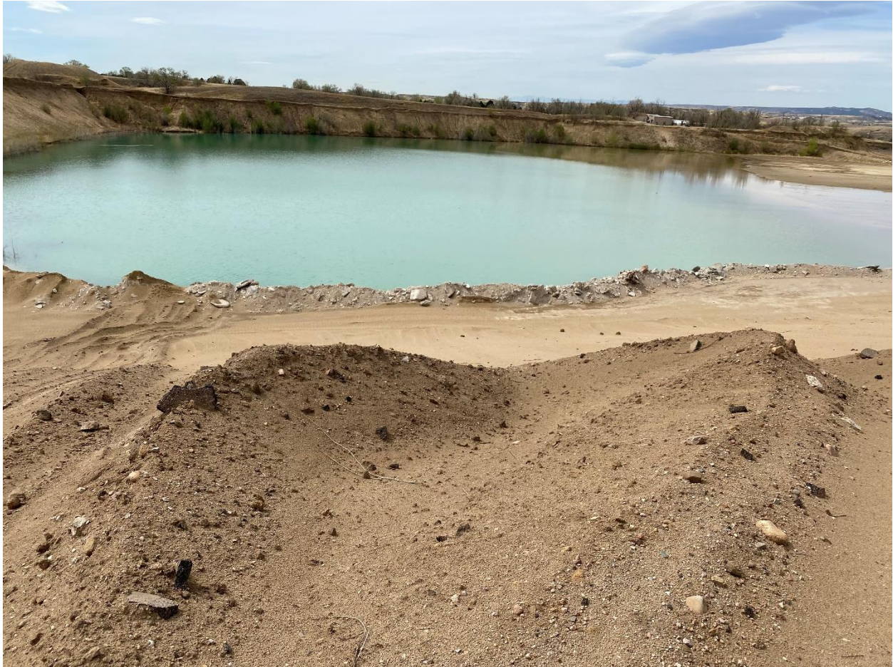
Photo 9. Butress slope looking south, area needs regrading
