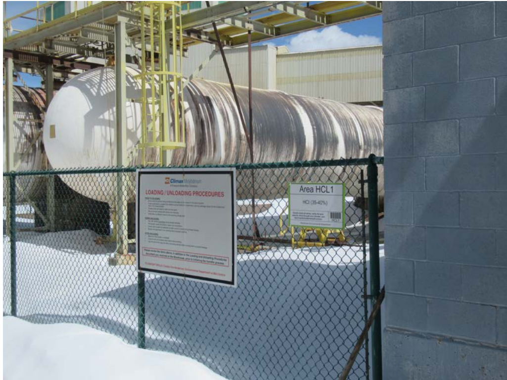
Hydrochloric Acid Storage Tank (1 of 2) and Sign
