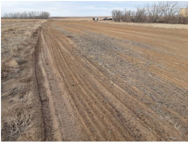
Haul Road where compaction was severe has been ripped. Spots with adequate vegetation was left undisturbed.
