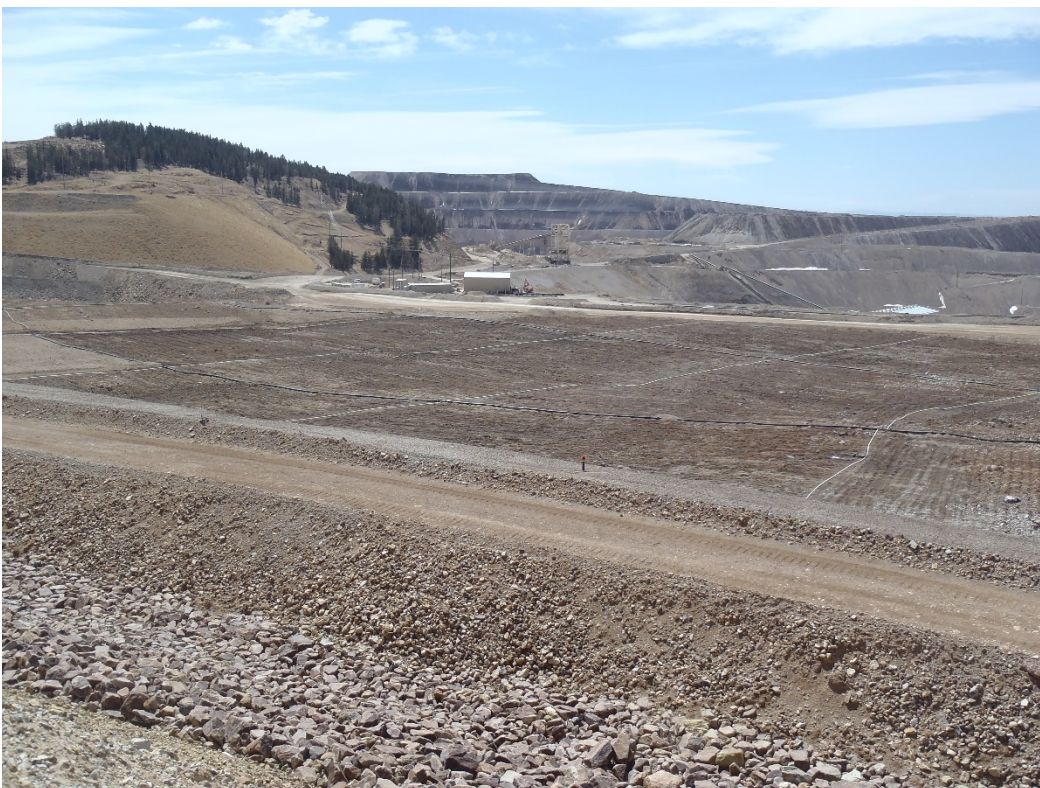
Photo 7. VLF2 leaching – no observed ponding (looking south from contractor buildings).
