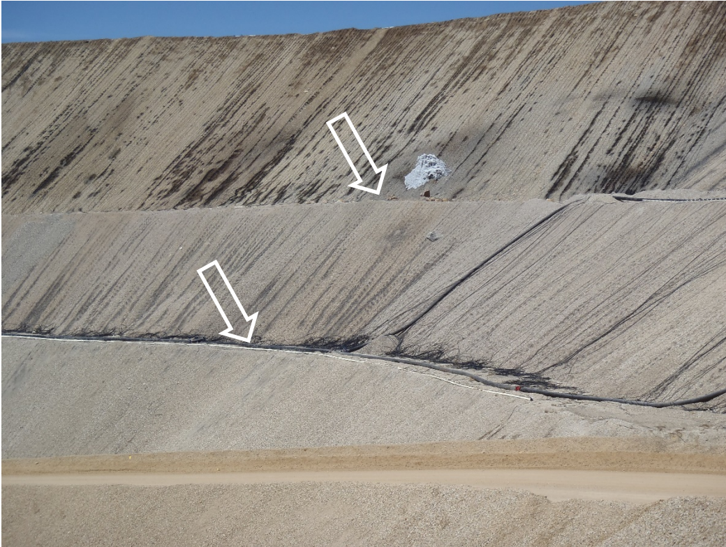
Photo 6. 10-foot benches/50-foot lifts on VLF2 above the HGM (looking NW from projects office).
