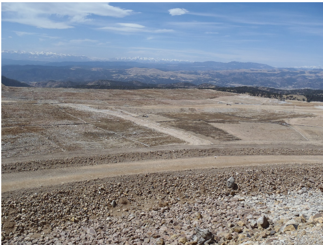
Photo 8. VLF2 leaching – no observed ponding (looking west from contractor buildings).
