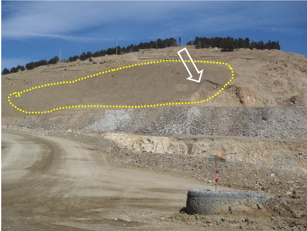
Photo 2. Growth media stockpile #32 (circled), sloughing (arrow) (looking NW).
