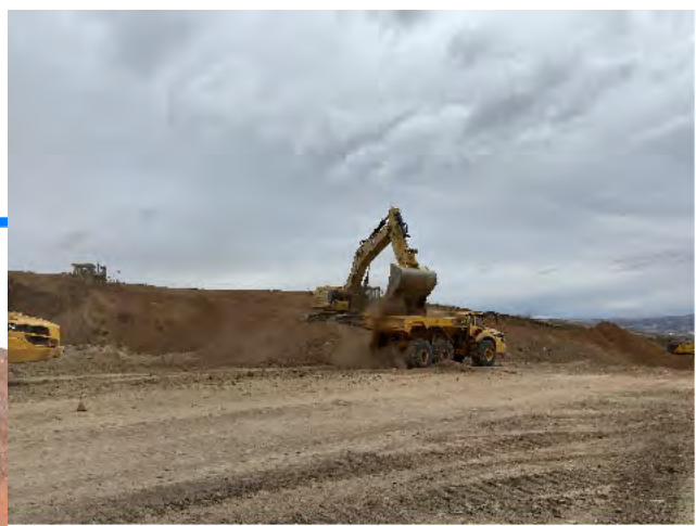
4. Excavator, dozer and haul trucks at borrow area
