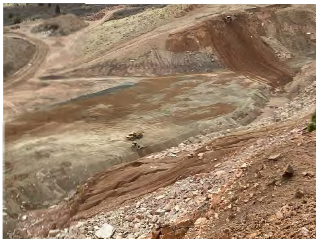
6. Dozer pushing material at south borrow area.
