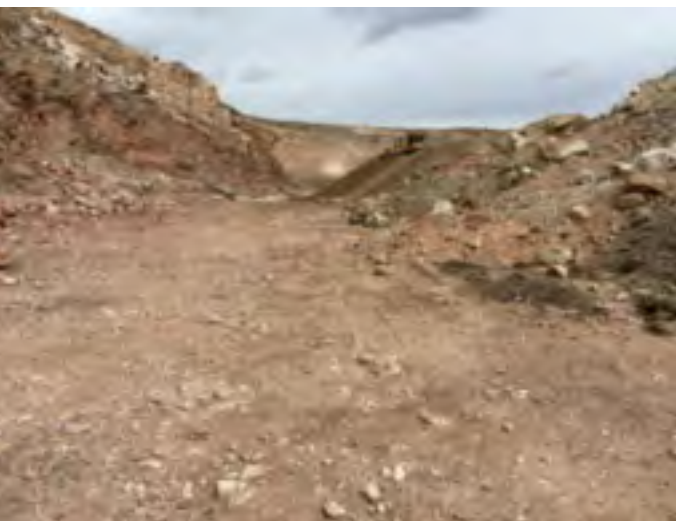
1. Safety buffer between toe of slope and work area.
