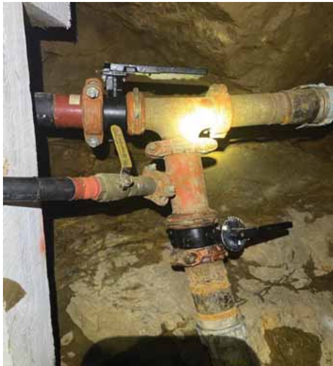
Figure 9 Cross Winze Valve Upgrade
