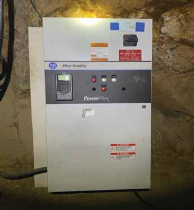
Figure 8 Cross Winze Pump VFD/Enclosure and Cross Discharge Meter
