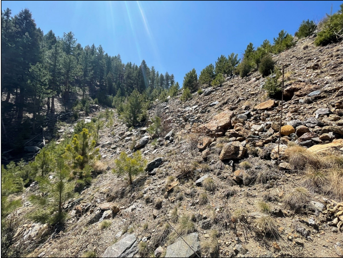
Figure 2. Broader view of the east-northeast facing CCP fill slope. Notice the junction with undisturbed ground and mature evergreens to the volunteer reclaimed CCP fill slope. View looking south.
