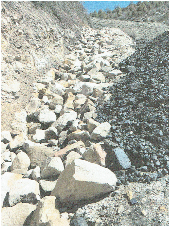
Pic. 4 – Encroachment of lower waste pile to clear water ditch.
