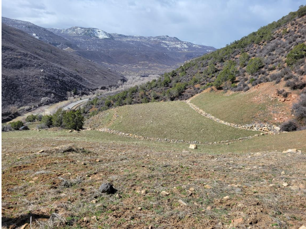
figure 9 – II west reclaimed topsoil pile in the foreground looking west with the II west reclaimed fill in the background outlined by constructed drainage channels.
