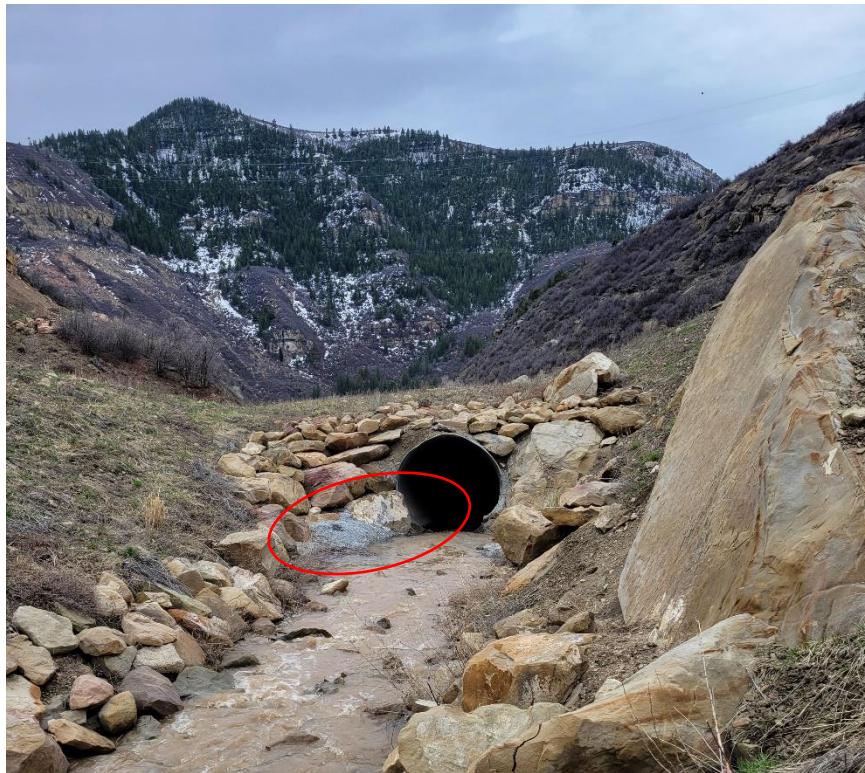
figure 4 – Mitigation of culvert undercutting with concrete on the upper portion of the reclaimed Elk Creek channel.
