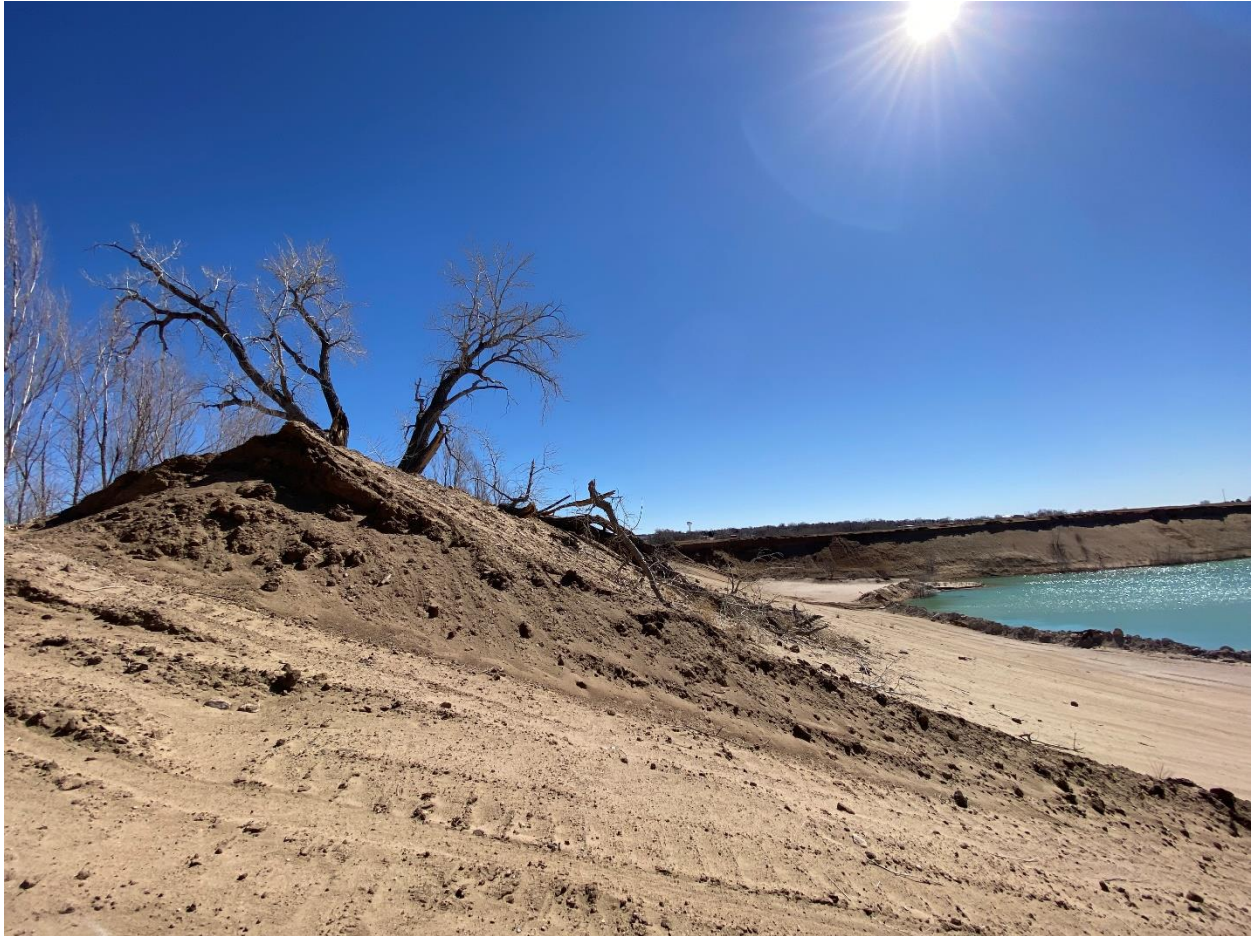
Photo 10. Buttress slope looking east, fallen tree within stockpiled material and buttress slope
