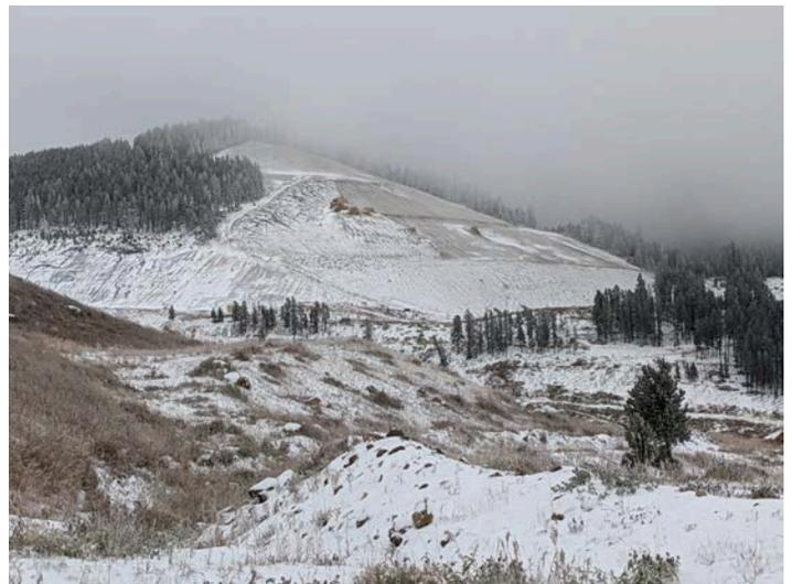
The laydown area above the Tie Camp Rock dump has been regraded and reseeded. The reclamation work looks good. No problems were noted.
