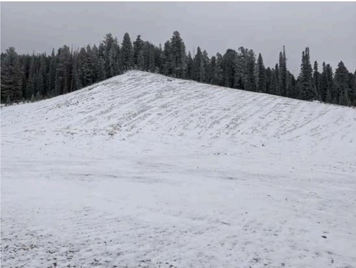
South Pit: Reclamation grading at the South Pit Landslide Crest Mitigation Area has been completed. The area was reseeded in the fall. The work observed appears to be in accordance with the approved reclamation plan. No problems were noted.
