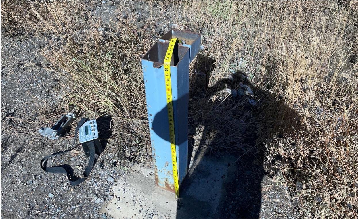
**Photo 3: Stickup of casing, measured from concrete base**
