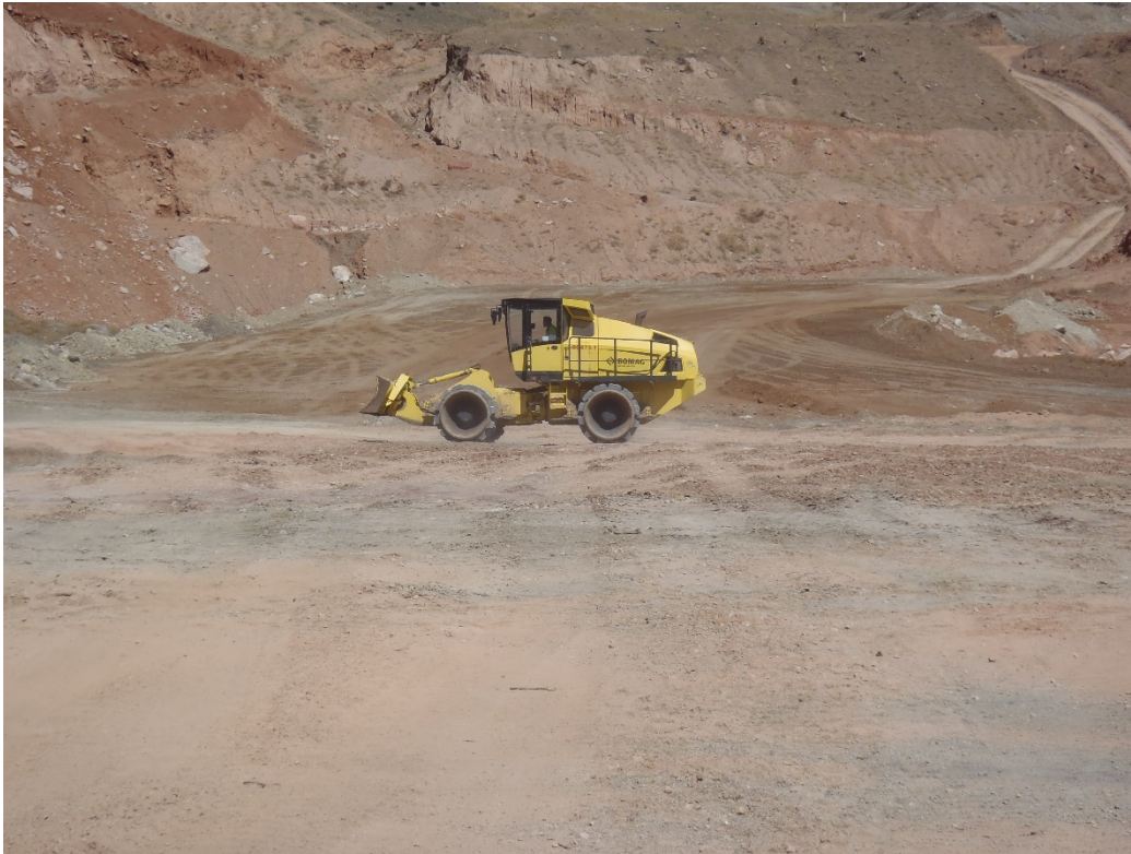
Photo 6. Compactor working latest lift (looking north from pit floor).
