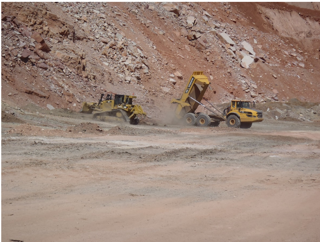
Photo 7. Dozer and haul truck working perpendicular to slide area.
