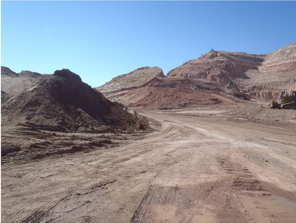
Photo 4. Excavation and hauling from the south end (looking south from future toe of slope).
