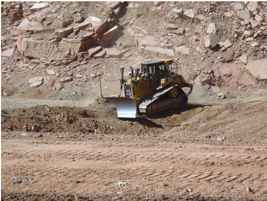
Photo 5. CAT D6 with GPS controls grading for lift thickness.
