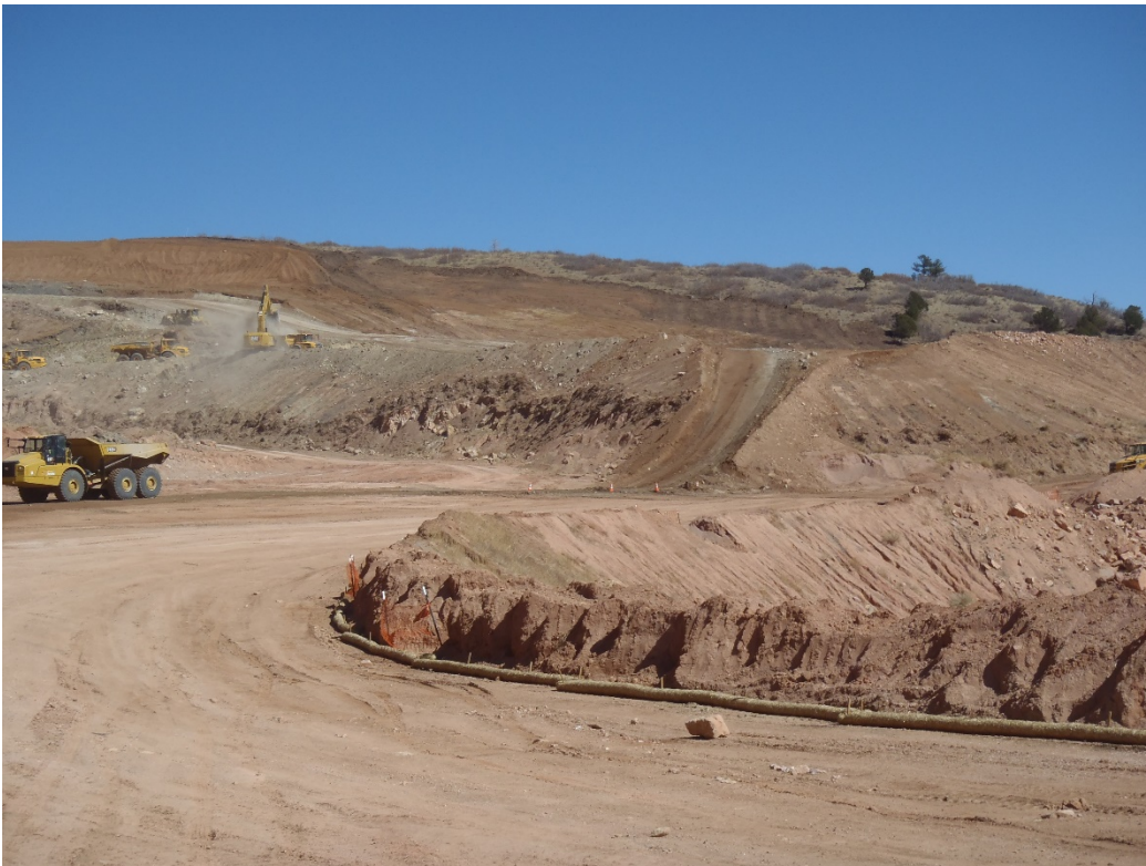
Photo 3. Excavation and hauling from the north end (looking north from future toe of slope).
