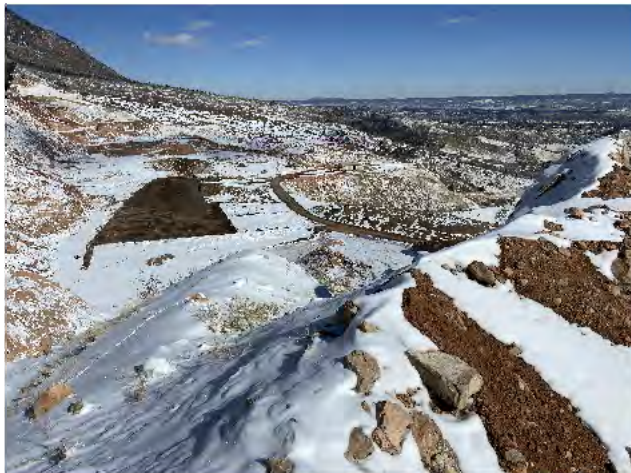
7. Material in pit is being spread by dozer. Snow was removed prior to placing fill.
