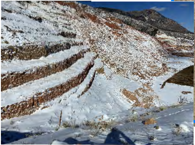
8. Reclamation benches on south-end.
