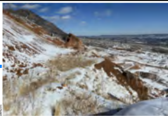
4. Large section of slide on the slope.
