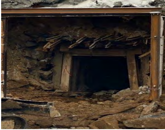
The collapsed Idaho tunnel entrance being excavated and cleaned up
