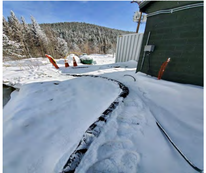
Figure 11 Treatment System Discharge Pipe and Intake Hose
