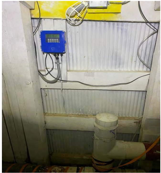
Figure 8 Cross Winze Pump VFD/Enclosure and Cross Discharge Meter
