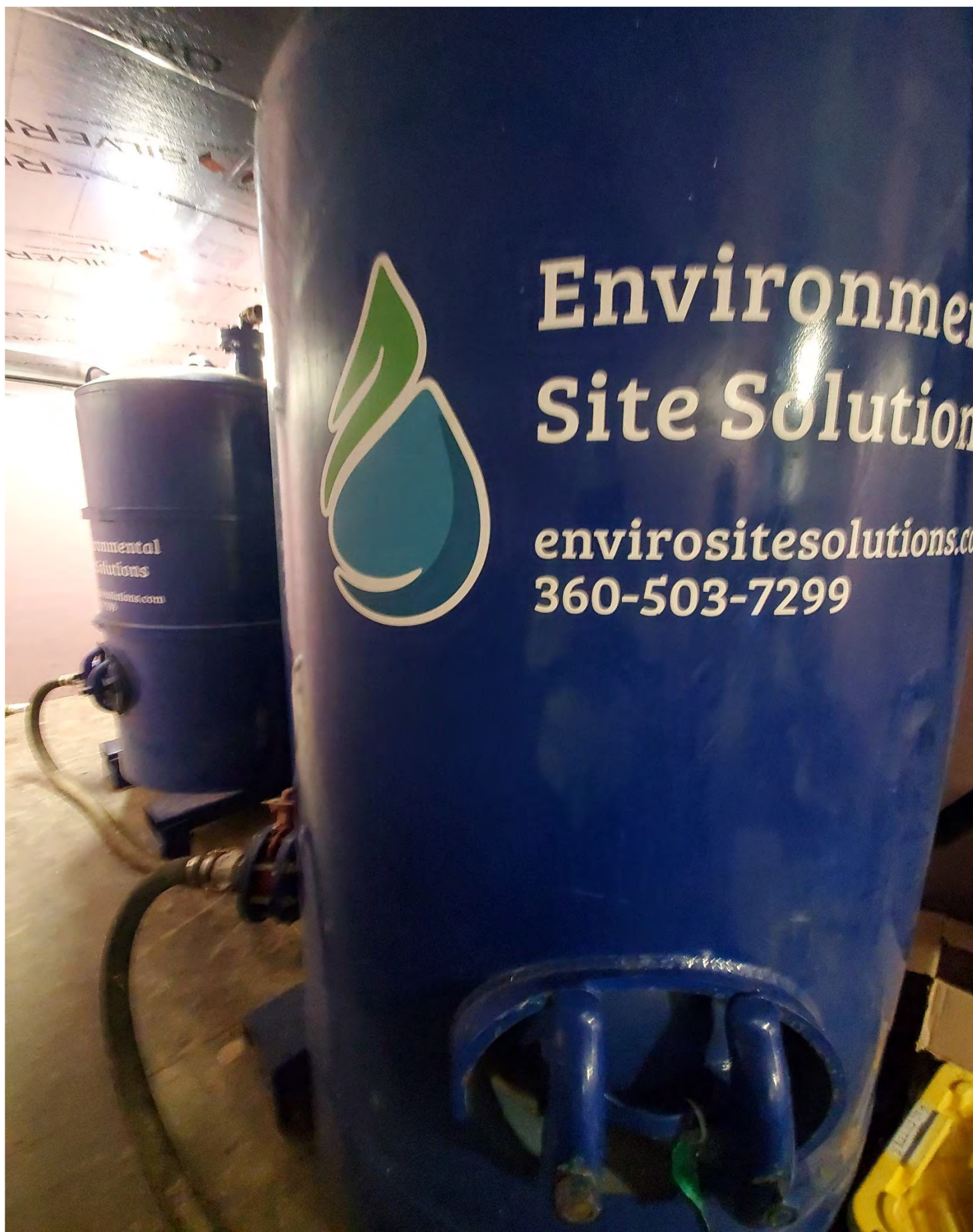
Figure 13 Vessels (provided by ESS) housing Metsorb Adsorptive Media (provided by Graver)
