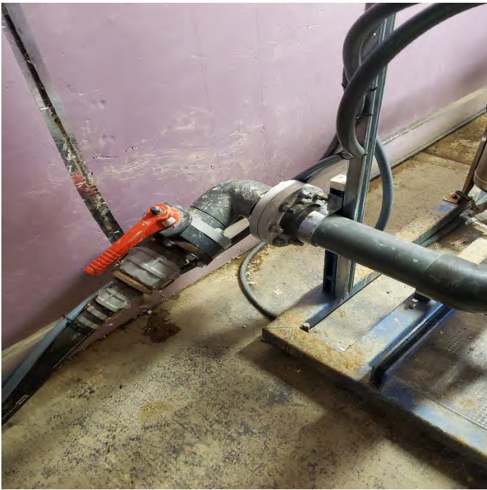
Figure 14 Isolation Valve and Backwash Tank
