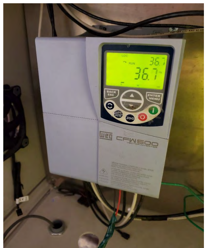
Figure 15 Programmable Logic Center (PLC) and Variable Frequency Drive (VFD)
