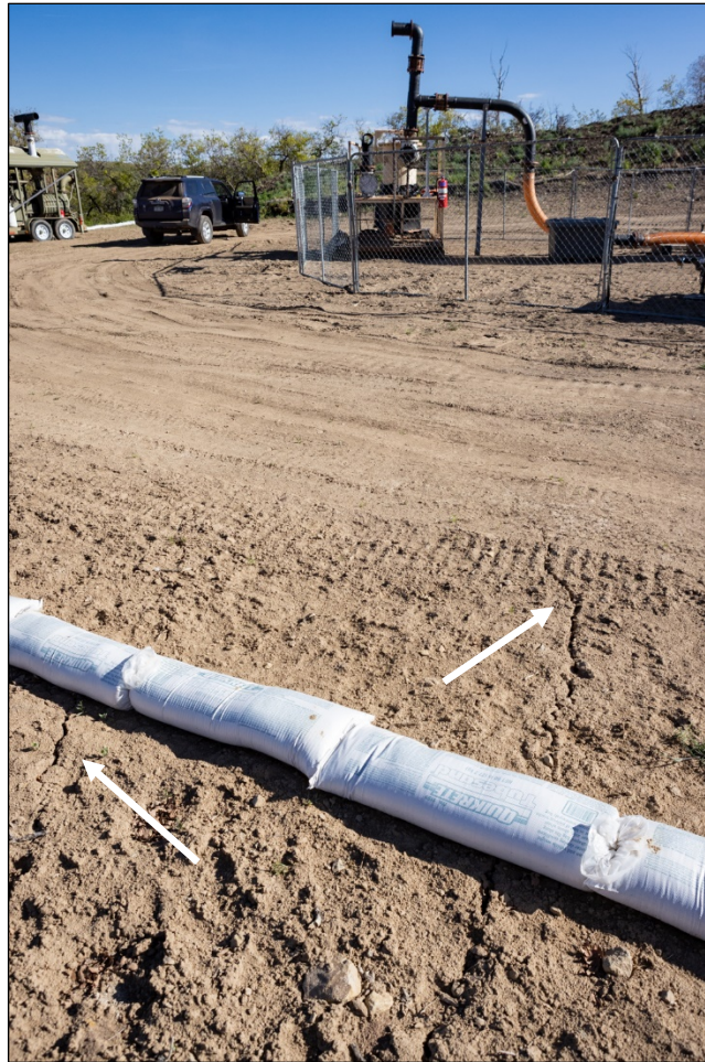
Figure 6. Northward view during the spring 2021 field visit of two smaller subsidence cracks (see white arrows) on the southern portion of the MVB SS1-6 pad.
