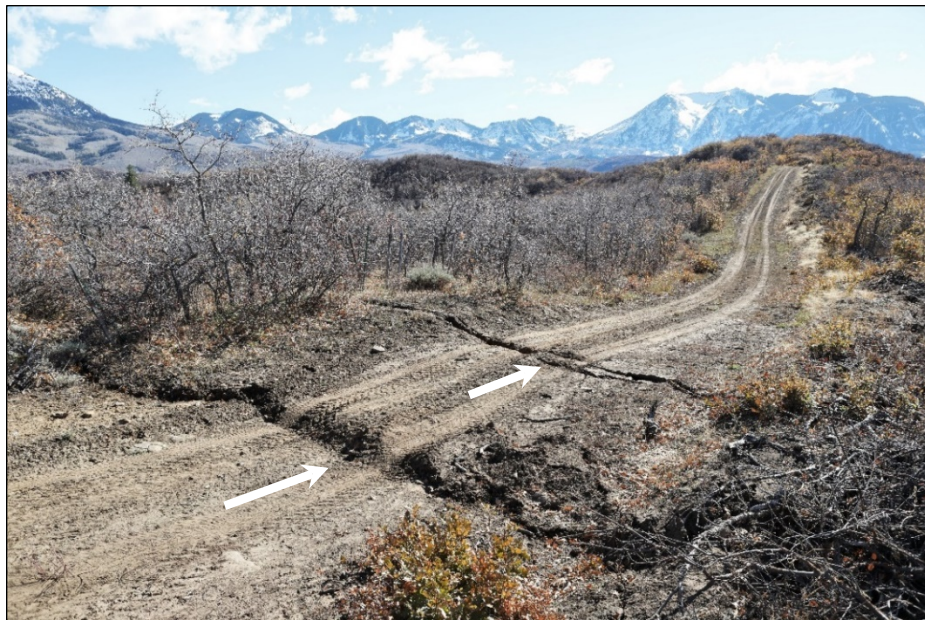
Figure 1. Fall 2018 southeastward view two parallel subsidence cracks (see white arrows) that appeared as a result of recent longwall mining beneath the area. Crack edge features suggested the two cracks were created at different times.
