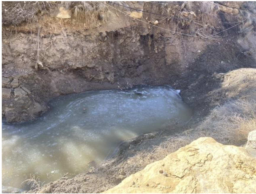
Photo 2: The last sump along the haul road before the sediment pond.
