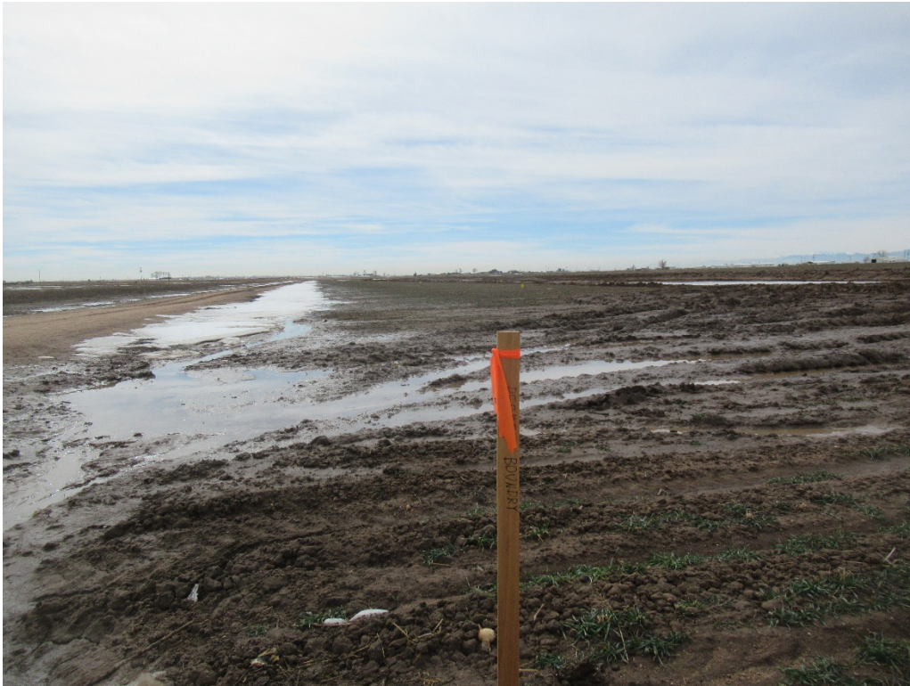
View of the typical permit boundary survey stake
