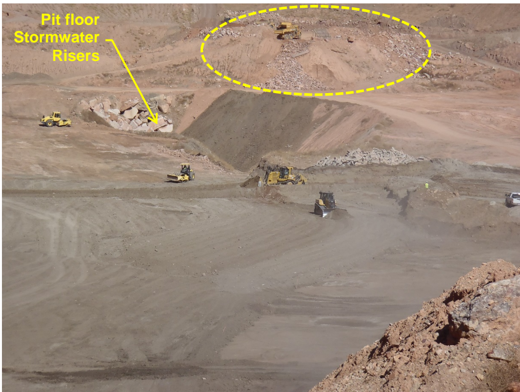
Photo 2. Backfilling operation (looking north at onsite "peninsula area" borrow).
