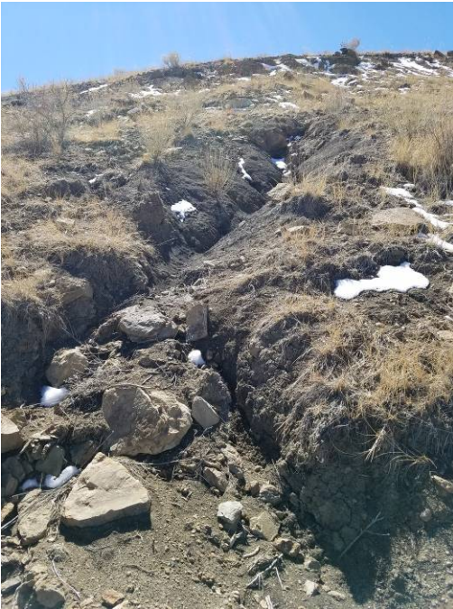
Figure 4. Rill above ditch D11.
