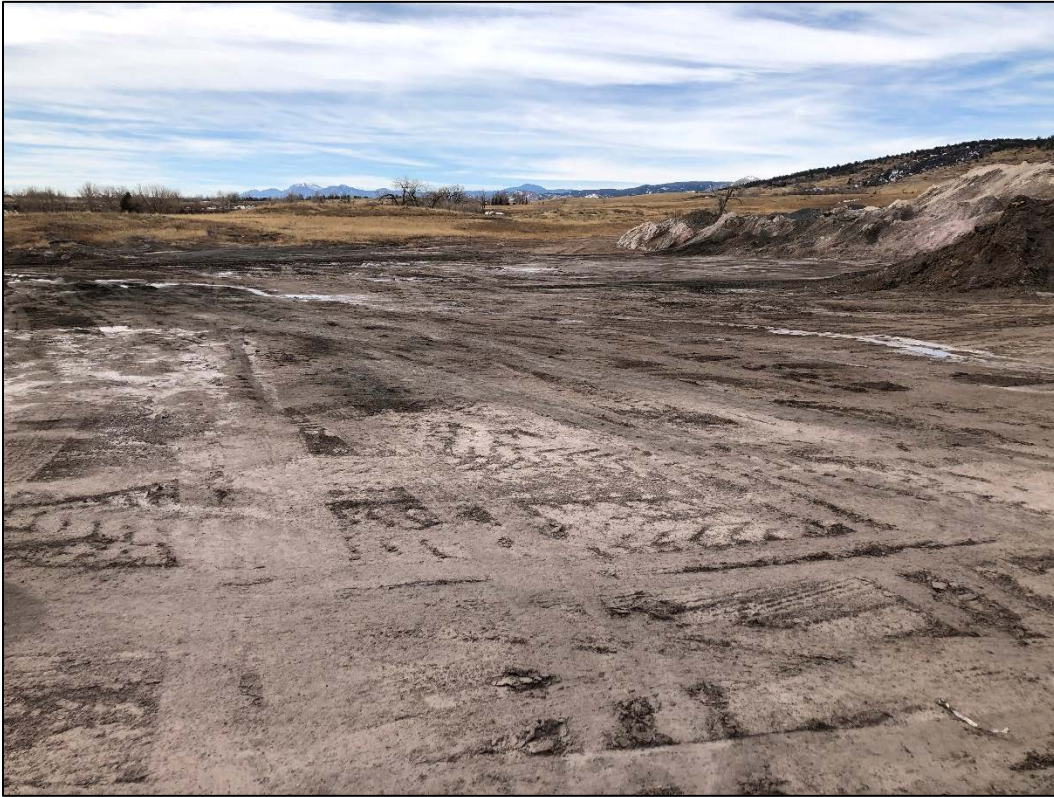
Photo 5. View looking south across southwestern portion of Pit C which has been backfilled with CKD but not yet capped with shale and clay material.
