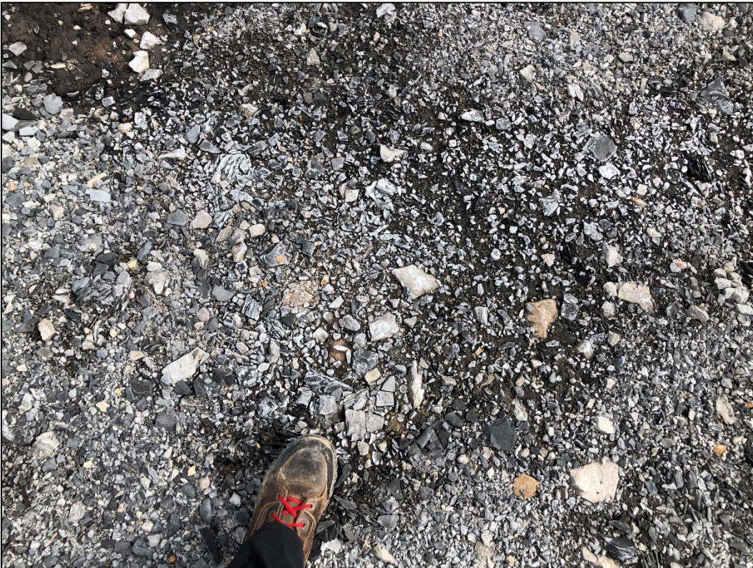
Photo 10. Ground view of shale and clay cap placed on backfilled portion of Pit C.
