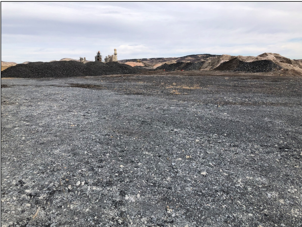
Photo 8. View looking north across southwestern backfilled portion of Pit C which has been capped with shale and clay material.
