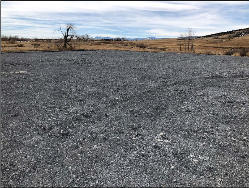
Photo 9. View looking south across southern backfilled portion of Pit C which has been capped with shale and clay material.
