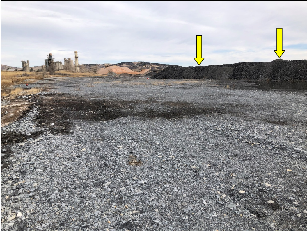
Photo 7. View looking north across western backfilled portion of Pit C which has been capped with shale and clay material. Note additional capping material (indicated) stockpiled in this area for future use.
