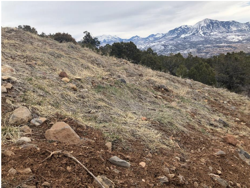
Stable slope below haul road (southwest corner of East Mine) with roughened surface to prevent erosion
