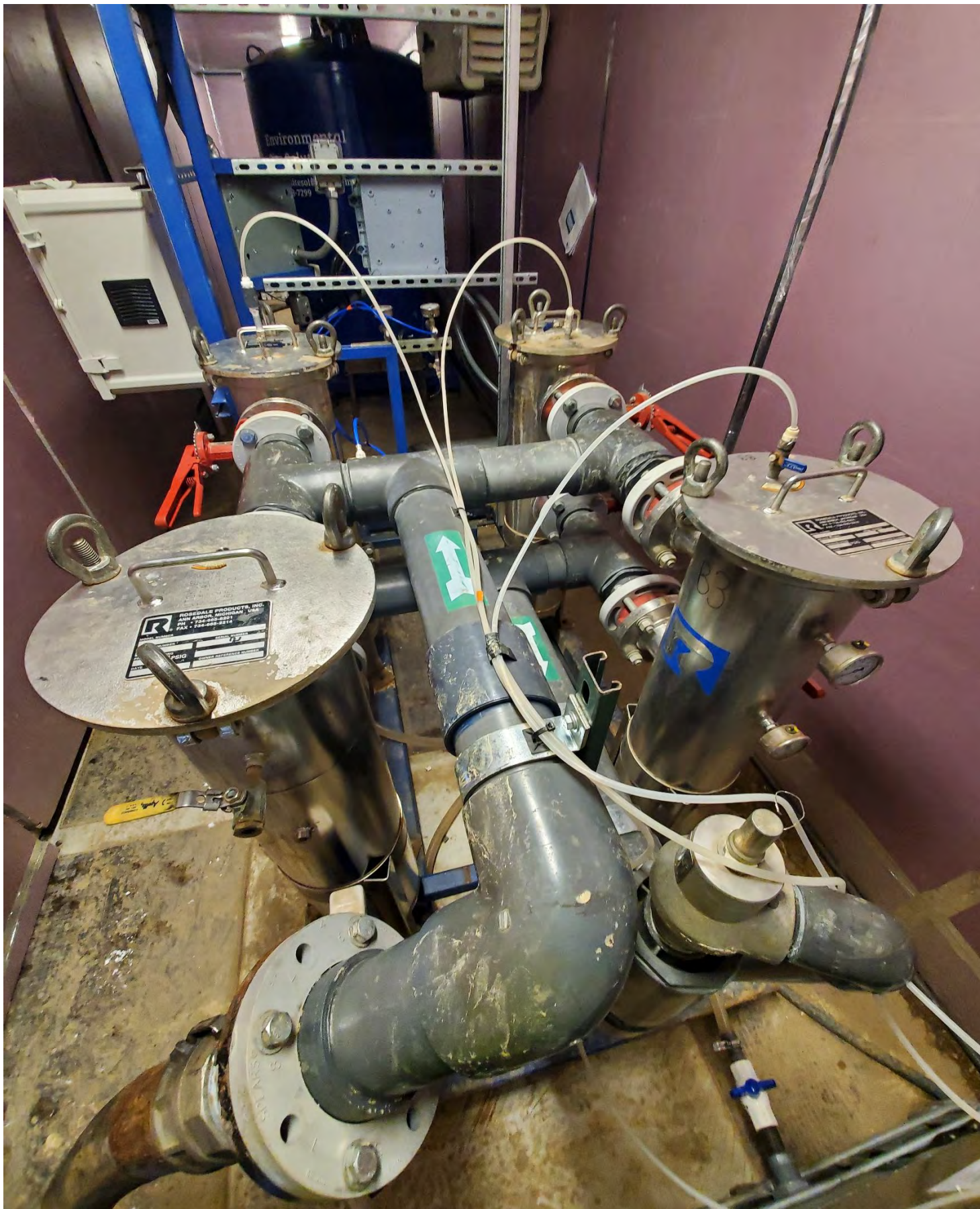
Figure 12 Skid Mounted Filtration System (provided by Ensero) 4 Stainless Steel Vessels – Housing 5-Micron Filtration Bags
