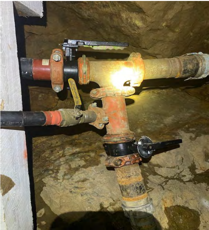
Figure 9 Cross Winze Valve Upgrade and XXX(Future Picture)
