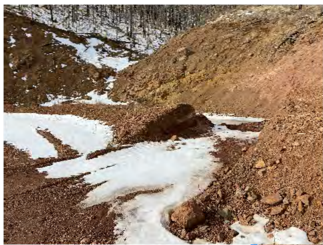
5. Level-control notch cut into pond.
