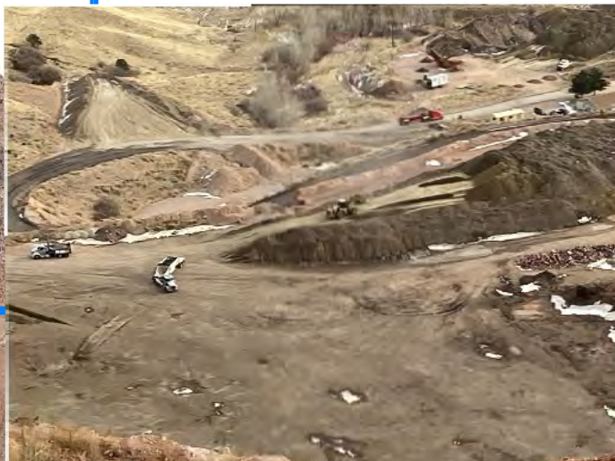
2. Topsoil stockpile at top of ramp being pushed by loader.
