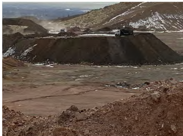
7. Fill material is dumped here then pushed by dozer.
