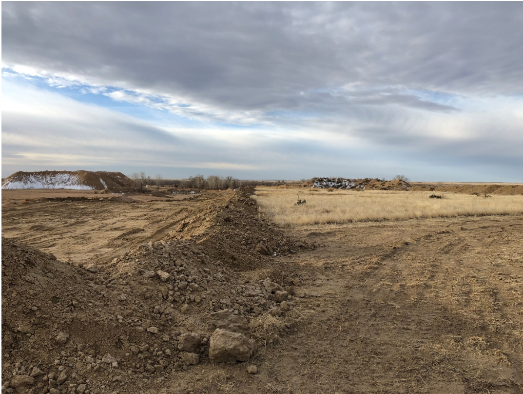
Photo 6: Topsoil being salvaged ahead of mining
