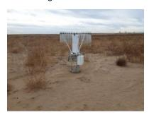
Weather station inspected. Minor erosion around concrete base. Divert sheet flows during revegetation cross ripping.
