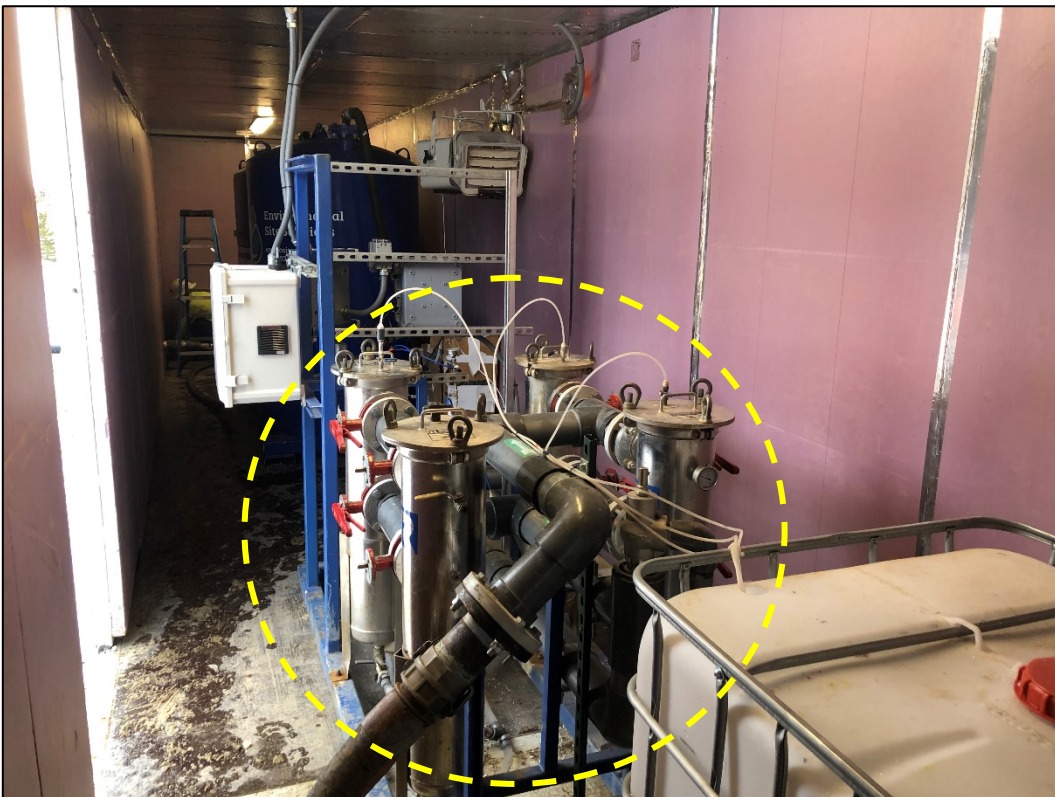
Photo 4. View inside insulated Conex box stored at Cross Mine, which houses new water treatment system. Note filtration system in foreground (circled) consisting of four bag filters, through which, mine water is first run.
