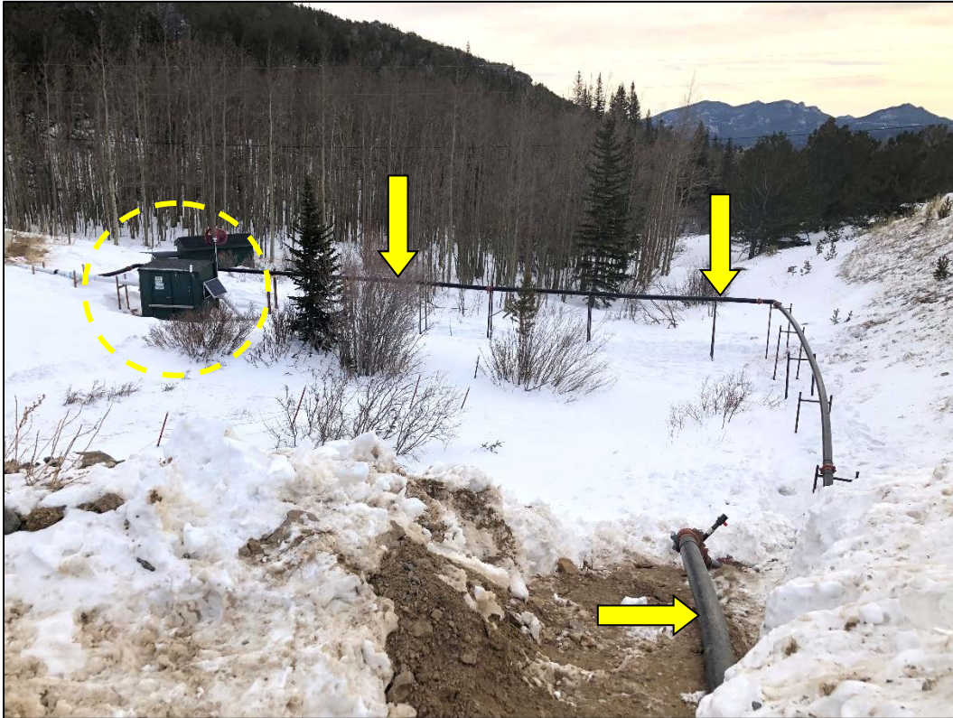
Photo 7. View looking east at new pipeline (indicated) installed to transport water from new treatment system to existing monitoring shed (circled) near Pond 2, where it joins with existing pipeline to discharge at permitted outfall on Coon Track Creek.
