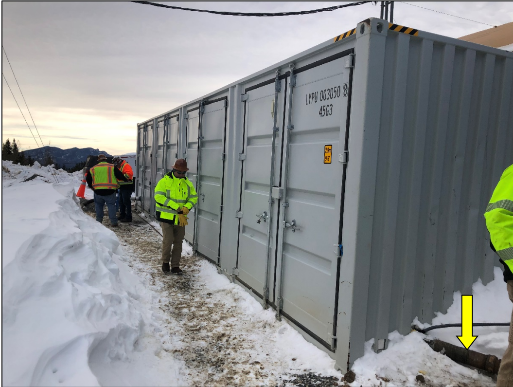
Photo 3. Closer view of insulated Conex box stored at Cross Mine, which houses new water treatment system. Note water inlet pipe (at bottom right, indicated) which transports mine water (from Pond 1) into treatment system.
