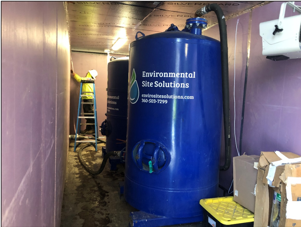
Photo 5. View inside insulated Conex box stored at Cross Mine, which houses new water treatment system. Note polishing system consisting of two blue vessels, through which, mine water is run after passing through filtration system. As mentioned above, only one of these vessels is in use at this time.
