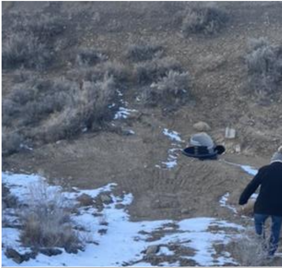
Photo 1: The completed maintenance at the site of the 016 Discharge Point. 016 is located in the gray upturned culvert. The Valve for 016 is located in the upturned black culvert.
