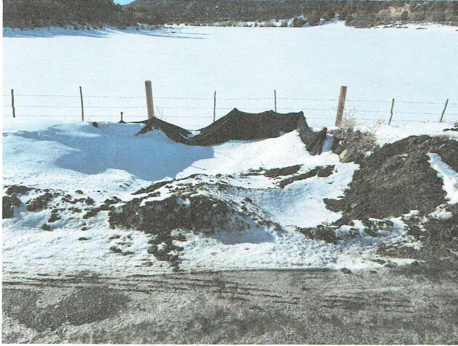
Pic. 3 – Snow removal bermed/built up in front of sediment traps.
