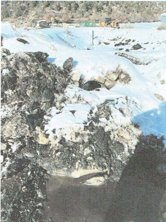
Pic. 4 – Culvert pipe to east detention pond blocked by snow removal operations.
