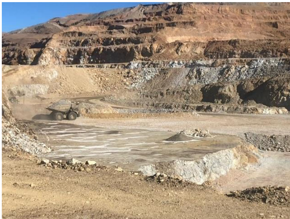
December 20, 2021 – High Compaction Backfill wheel rolling and leveling (GF)
