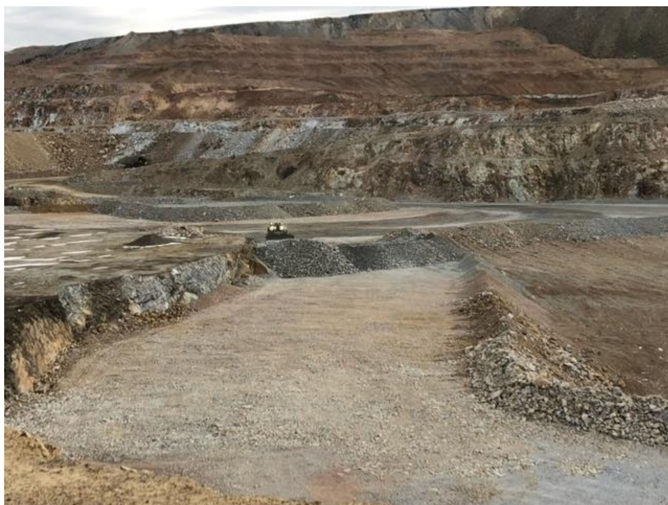
December 21, 2021 – High Compaction Backfill placement (GF)
