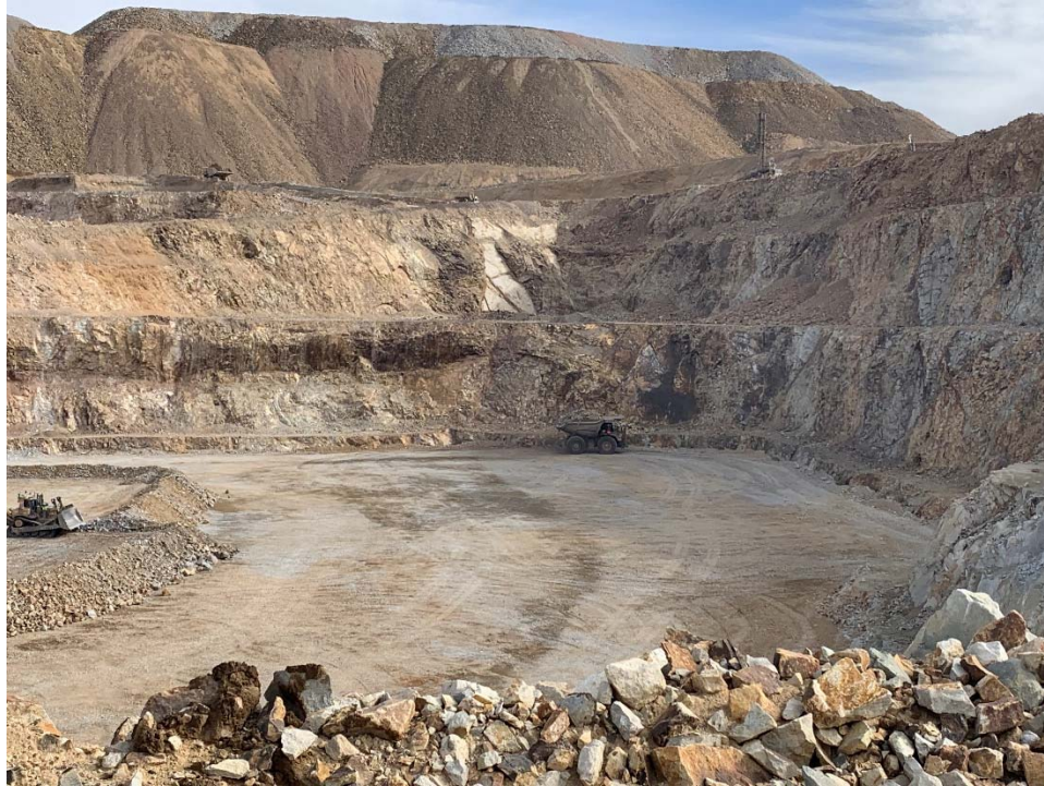
November 18, 2021 – High Compaction Backfill wheel rolling and placement (TW)
